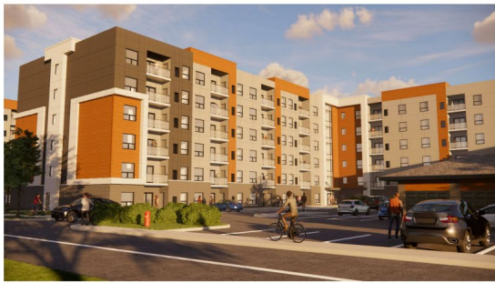
FRONT - NORTH WEST CORNER
