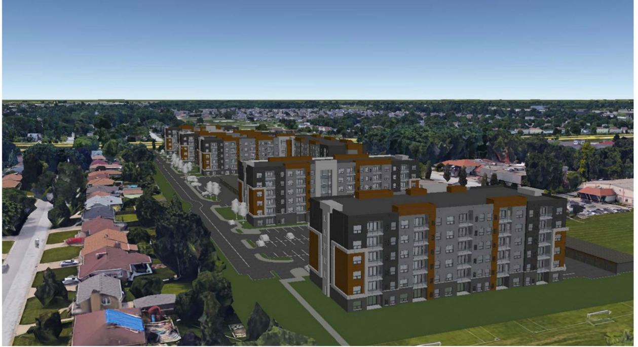
FIGURE 8 – SITE AERIAL VIEW – NORTH-EAST CORNER
