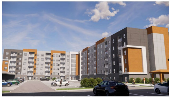
FRONT - NORTH WEST CORNER
