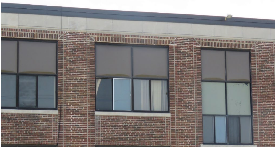
Stone parapet on roofline, now flashed with metal, and soldier and rowlock brick at glazing lintels.
