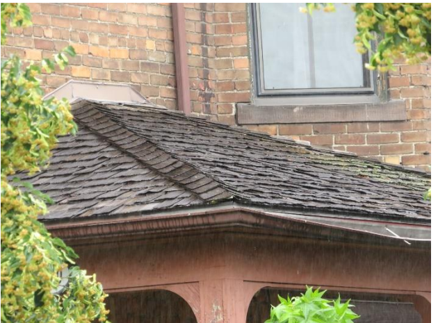
Photograph of the cedar roof and front dormers at the junction of both properties; and photograph of the cedar shingle roof over the side porch of 548-550 Devonshire Road
