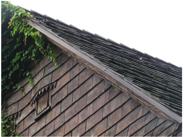
Various close-up photographs of the cedar wood shingle roof and gable ends from the rear of both properties
