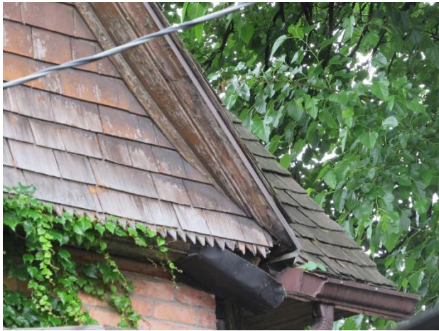
Various close-up photographs of the cedar wood shingle roof and gable ends from the rear of both properties
