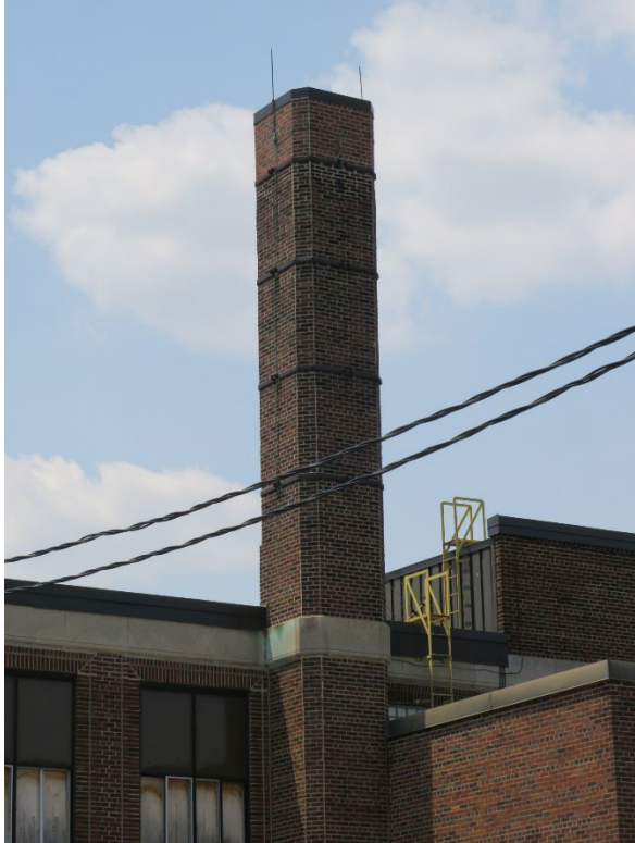
Square brick chimney with chamfered corners
