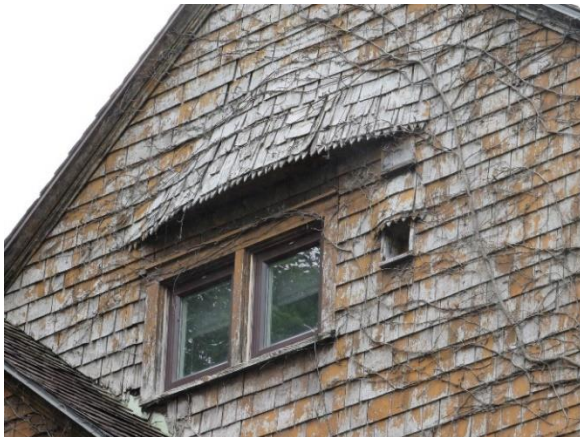
Close-up of the wood shingle siding and “dragon teeth” edging details on the north (side) gable face of 546 Devonshire Road
