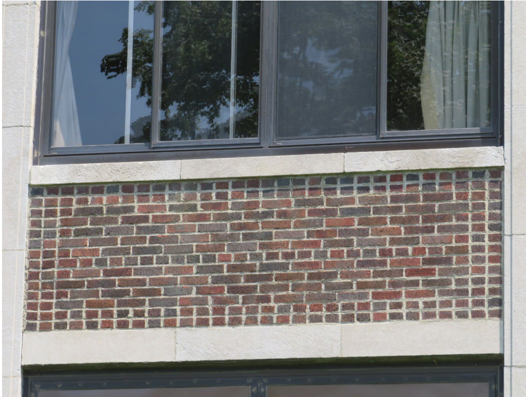
Typical brick panel featuring variety of header and stretcher brick between the floors.
