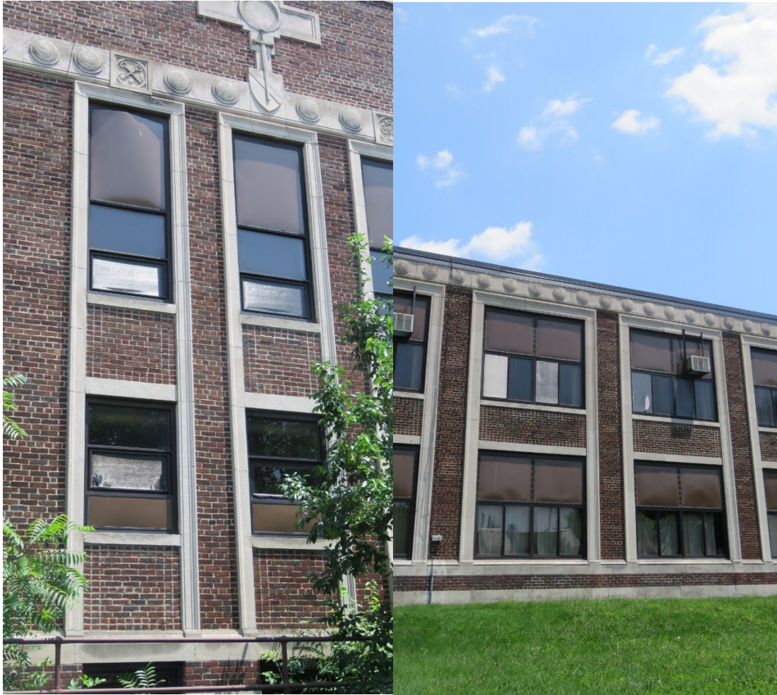
Bays of rectangular windows with stone frames (left) and squared windows with stone surrounds (right) on front facade
