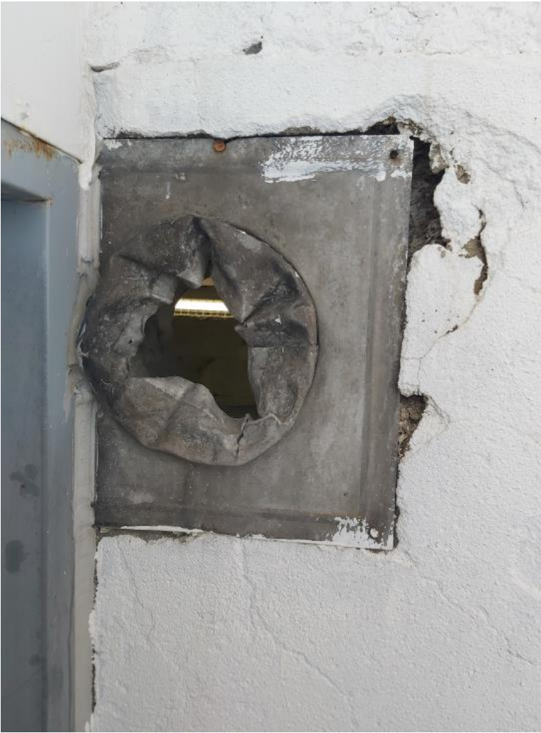
11. Defective exhaust system.
