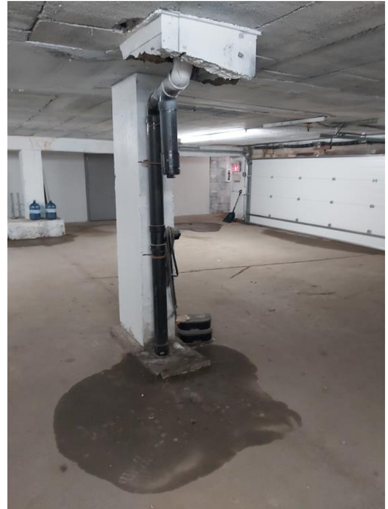
6. Water infiltration in underground parking garage.
