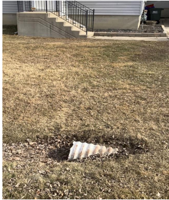
3726 Riberdy Road – 375mm diameter CSP pipe culvert with no observed deformation but rusted. Approximately 20% of this pipe was observed to be blocked with debris. No headwall was observed for this culvert.
