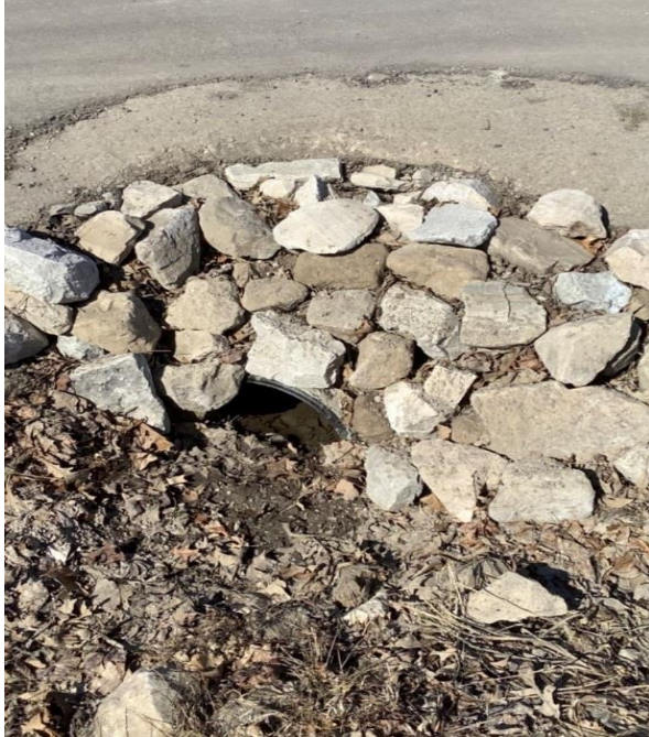
3697 Turner Road – 300mm diameter CSP pipe culvert with no observed deformation and rusted. Approximately 70% of this pipe was observed to be blocked with debris. The headwall consists of concrete and stone.
