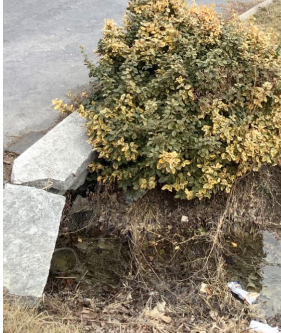
3923 Riberdy Road – 375mm diameter CSP pipe culvert with no observed deformation and rusted. Approximately 40% of this pipe was observed to be blocked with debris. The headwall is a mix of the asphalt driveway and the stone resting on top of it.
