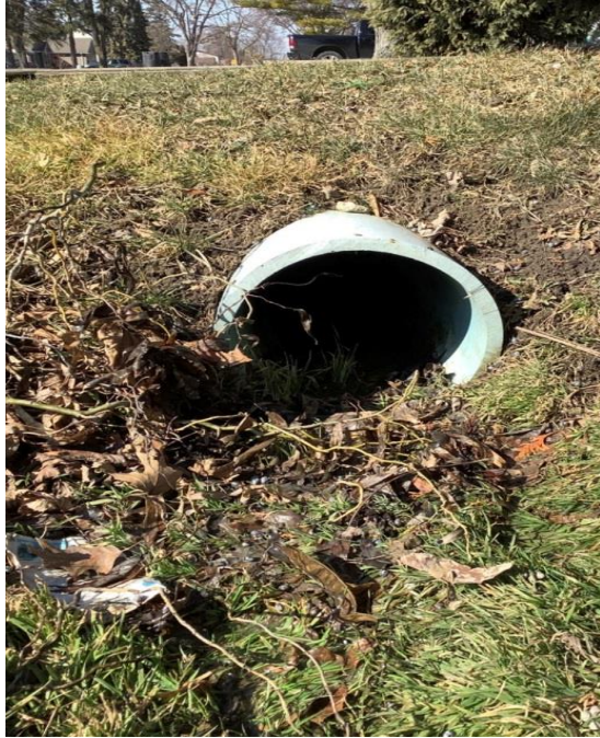
3860 Woodward Boulevard – 300mm diameter PVC pipe culvert that is in good condition with no observed deformation. Approximately 10% of this pipe was observed to be blocked with debris. No headwall was observed for this culvert.
