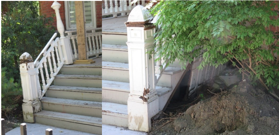
Photos of the newel posts, skirting, railings & guards.
