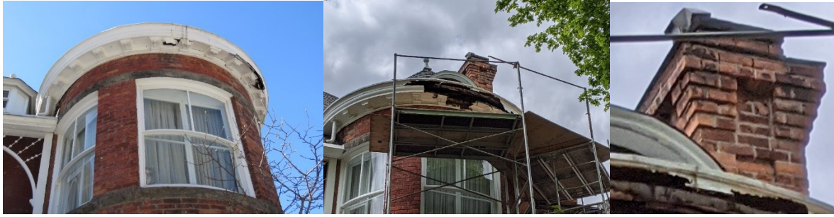
Before Photos of the turret and chimney
