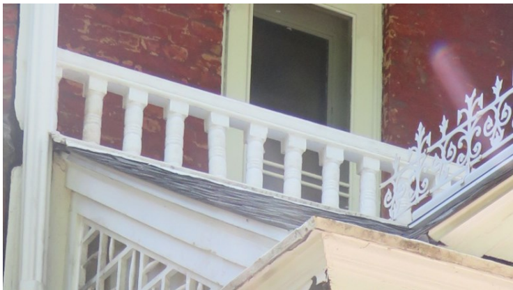
Current railings with similar design on 2nd floor balcony
