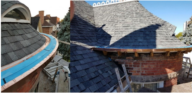
Repair work in progress
