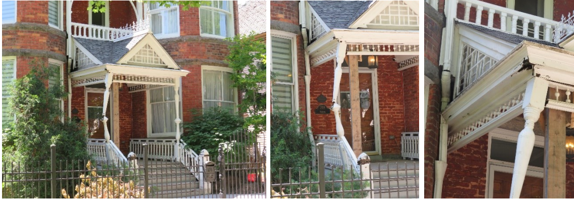
Photos of porch (taken June 2022)
