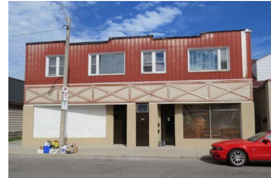
Figure 121. Example of a building where original brick has been covered
