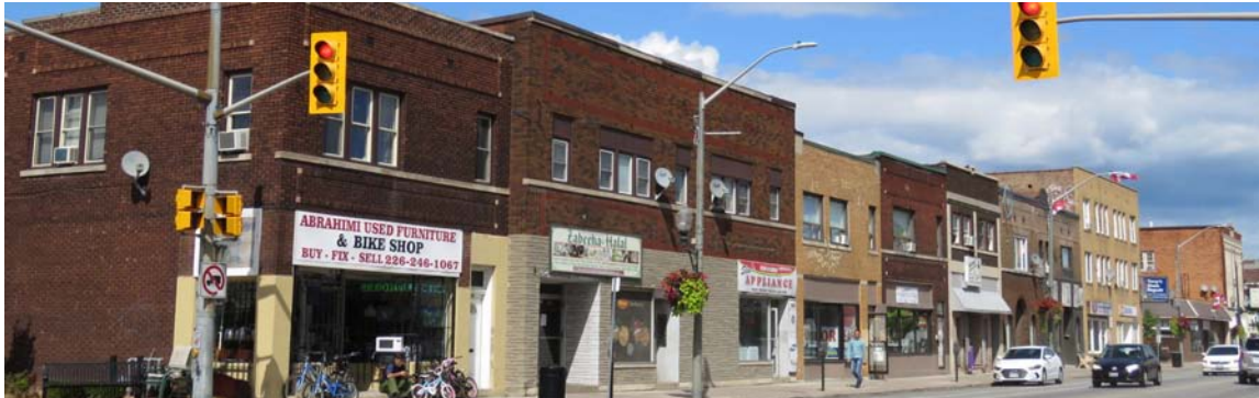
Figures 83. Buildings along Wyandotte Towne Centre BIA Mainstreet where most original architectural features, windows, and storefronts have been retained, creating good street presence
