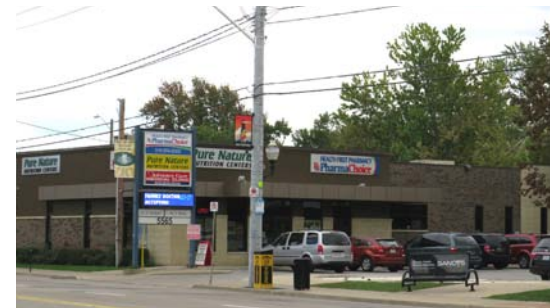
Figure 136. Non-traditional commercial built form, with parking at the intersection corner and an over-use of signage
