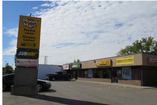
Figure 120. Gap in the street facade along Wyandotte Street East, Windsor
