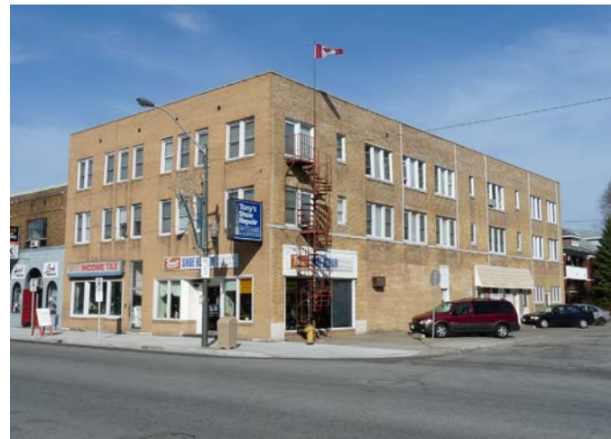
Figure 74. Leatherdale Block located at 1380-1394 Wyandotte Street East
