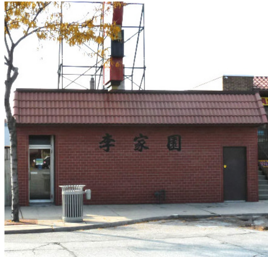
Figure 50. Avoid covering windows with wood or other materials (567 Pelissier Street)
