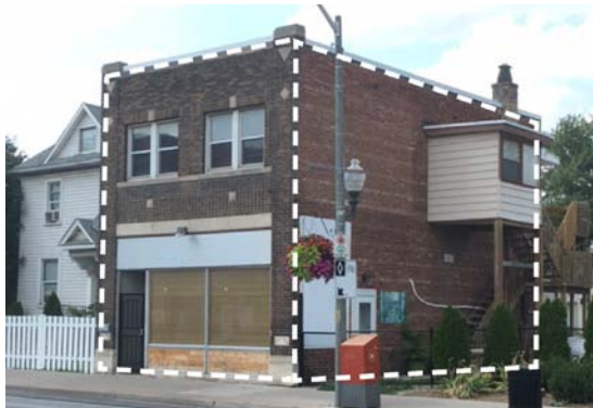
Figure 15. A typical storefront located on Wyandotte Street East
