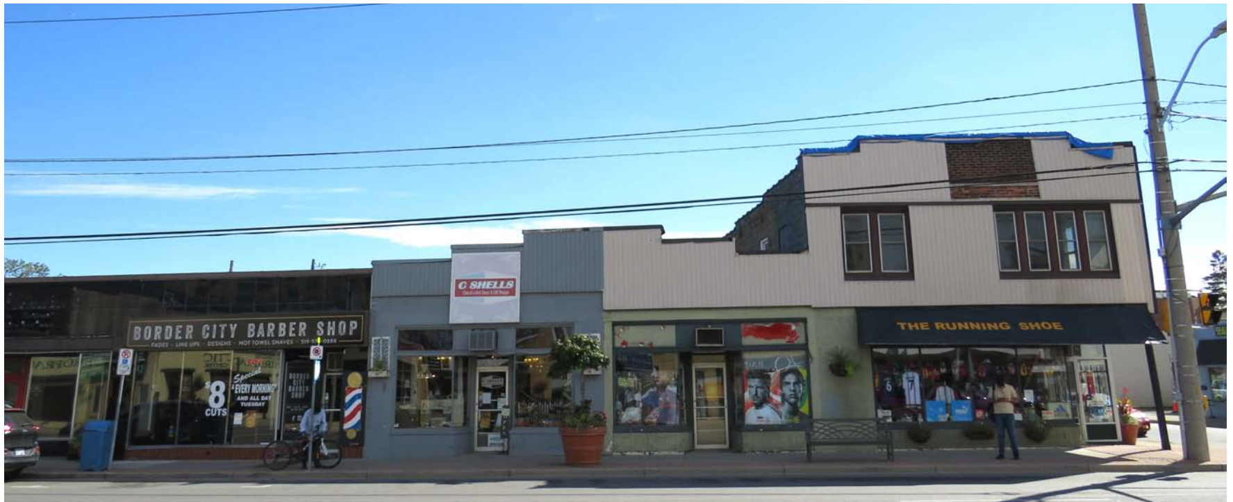
Figure 119. Building façades along the south side of Wyandotte Street East in the Pillette Village BIA, where aluminum siding covering the original brick
