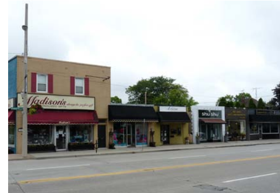
Figure 40. A continuous street wall is desirable such as this example along Wyandotte Street East in Olde Riverside
