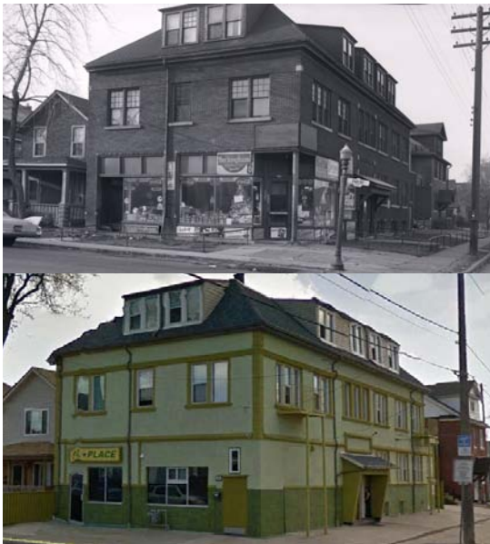
Figure 67. EFIS is an undesirable building material that is often used to cover brick
