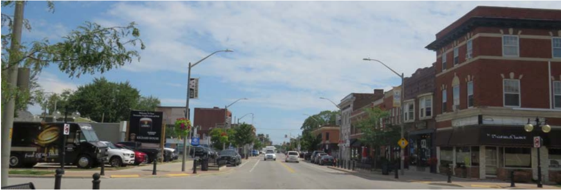
Figure 68. Commercial/Mixed-Use Infill Design Example located at the corner of Wyandotte St. E., and Windermere Rd. where a vacant site currently exists.
