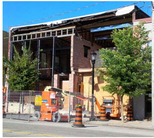
Figure 57. 3236 Sandwich Street during renovations
