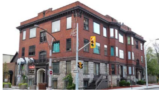
Figure 43. Traditional Main Street building on Park Street
