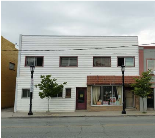
Figure 56. 3236 Sandwich Street before renovations, 2012
