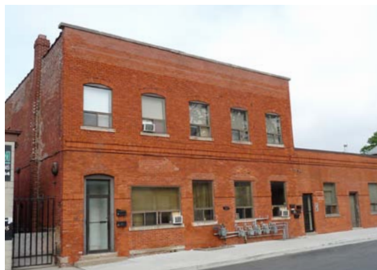
Figure 79. Langlois Street, Windsor
