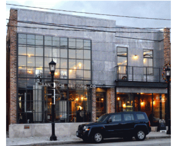
Figure 58. 3236 Sandwich Street at completion
