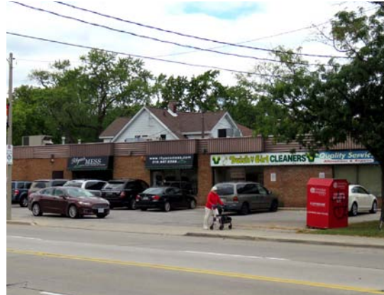
Figure 132. Gap in the street facade along Wyandotte Street East, Windsor
