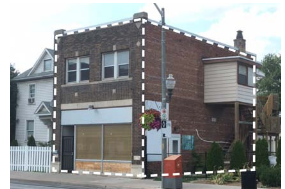
Figure 15. A typical storefront located on Wyandotte Street East
