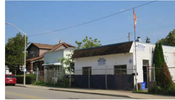
Figure 112. Example of a hodge-podge of building types and materials on the east side of Drouillard Road north of Metcalfe Street
