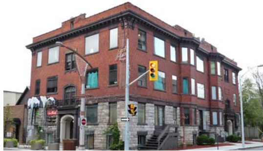
Figure 43. Traditional Main Street building on Park Street
