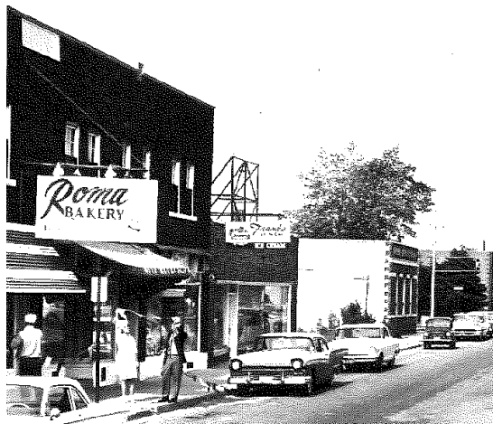
Figure 129 Traditional Main Street facades along Wyandotte Street East by St. Louis Avenue, date unknown (Fullerton)
