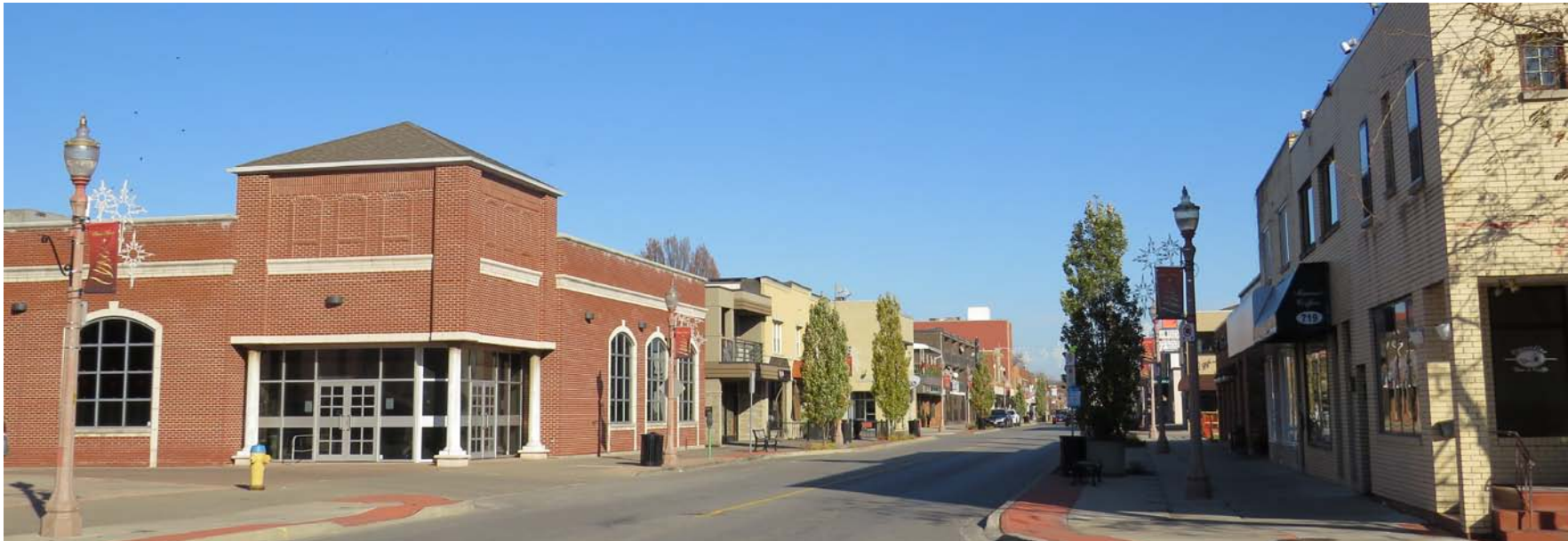
Figure 142. Erie Street East looking east from Louis Avenue
