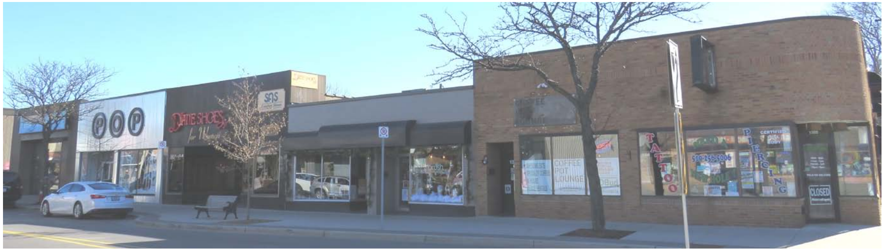
Figure 154. Building façades on Ottawa Street between Hall Avenue and Moy Avenue
