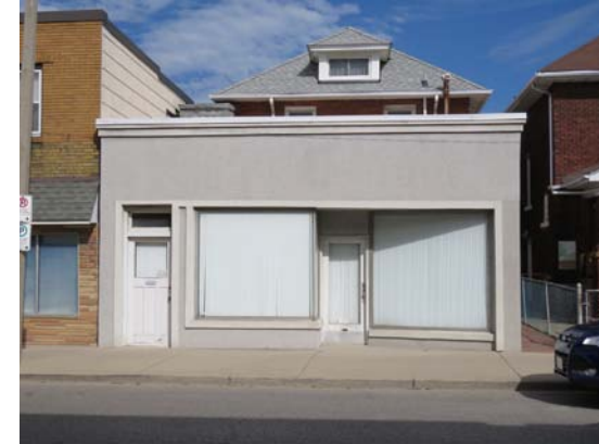
Figure 125. A traditional storefront has been covered with non-traditional material and windows have been covered
