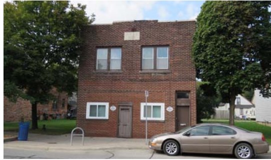
Figure 111. Example of a traditional commercial building that has doors and windows bricked in and replaced
