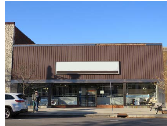
Figure 156. Windows are barred and non-traditional material covers the facade
