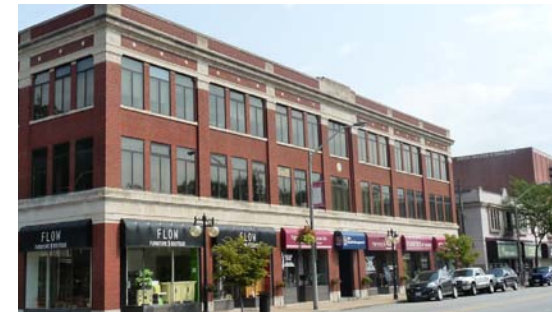
Figure 44. Traditional Main Street building on Wyandotte Street E
