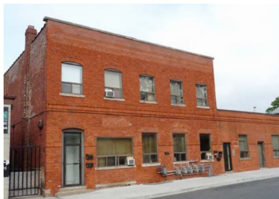
Figure 79. Langlois Street, Windsor
