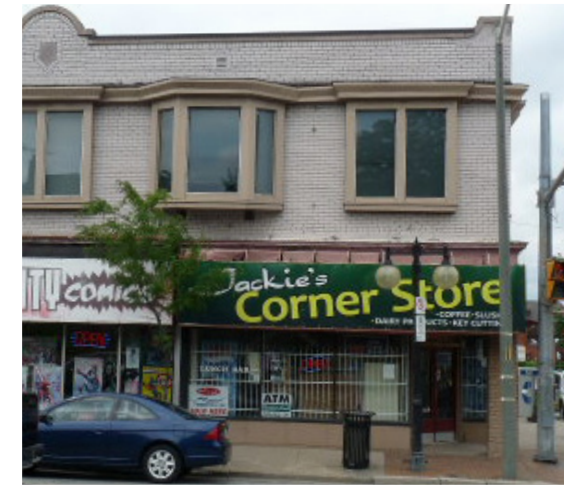
Figure 89. Security bars on windows make the area feel unsafe
