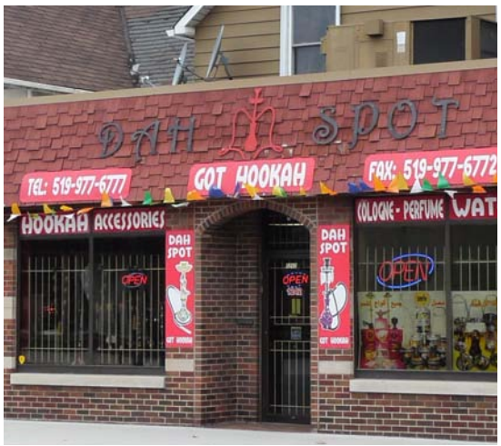
Figure 38. Bars over windows give the impression that the area is unsafe
