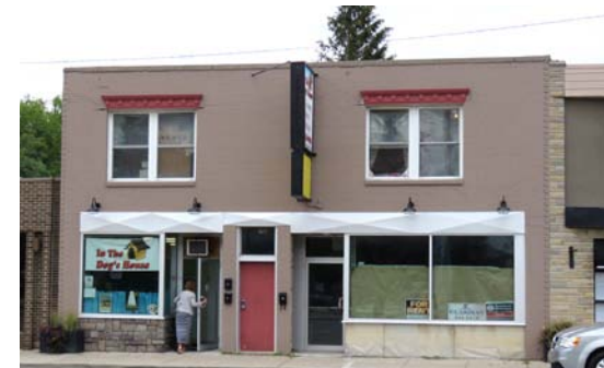
Figure 137. Original brick has been painted over, and non-traditional building materials have been added on top
