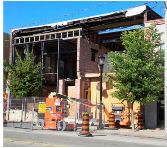
Figure 57. 3236 Sandwich Street during renovations
