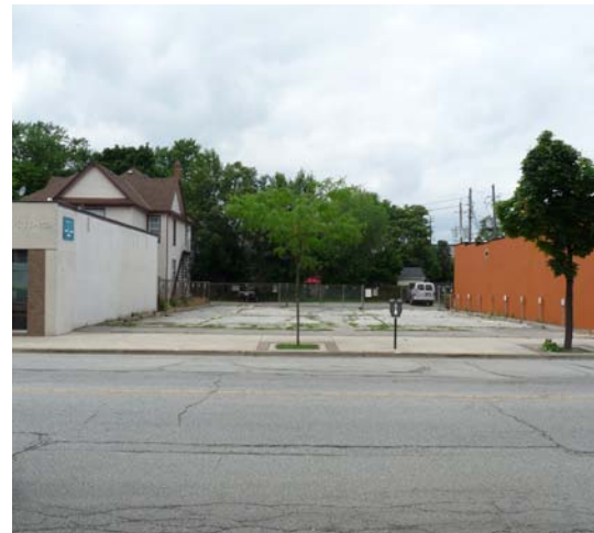
Figure 88. Gap in the street facade along Wyandotte Street East, Windsor
