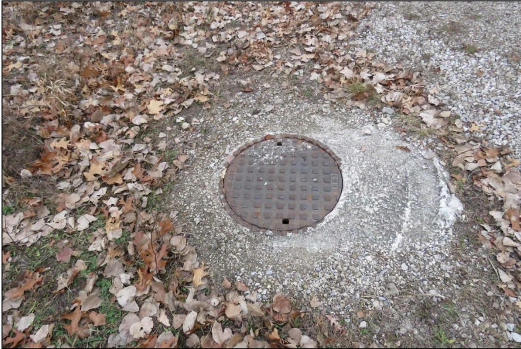
Figure 7 - Storm sewer manhole within Third Street right-of-way
