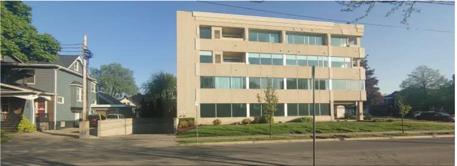
Photo 5: View of north wall and access to underground parking along Shepherd St.
