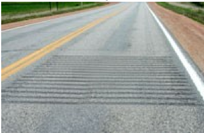
Figure 4: Transverse Rumble Strip Example (Source: Neal Hawkins/Iowa DOT)
