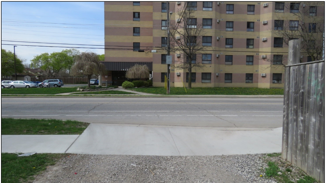
Figure 4 - Looking north towards College Avenue from alley (905 Bridge Avenue on right)
