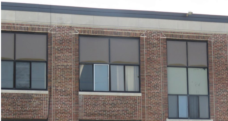
Stone parapet on roofline, now flashed with metal, and soldier and rowlock brick at glazing lintels.
