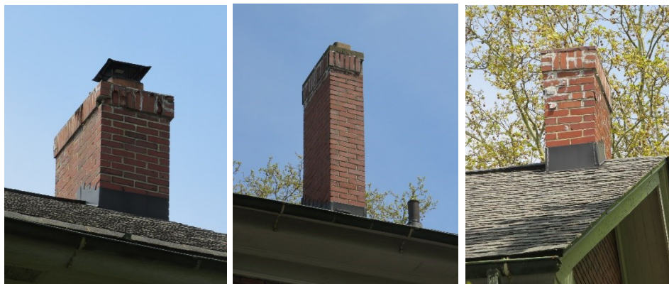
Photos of the three chimneys (taken May 8, 2023)
