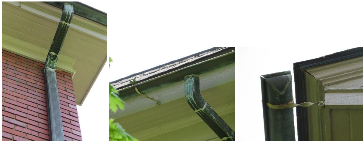
Photos of the gutter system (taken May 8, 2023)
