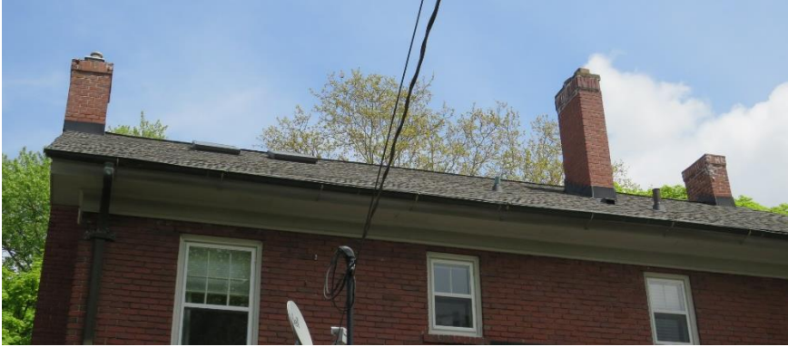
View of the three chimneys from the rear yard
