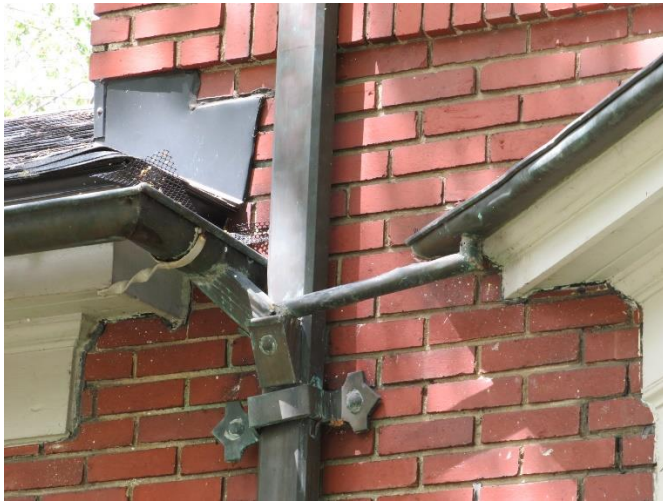
Close-up views of the downspouts, brackets, and connections
