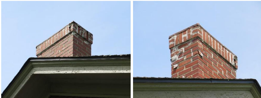
Close-up views of the south chimney
