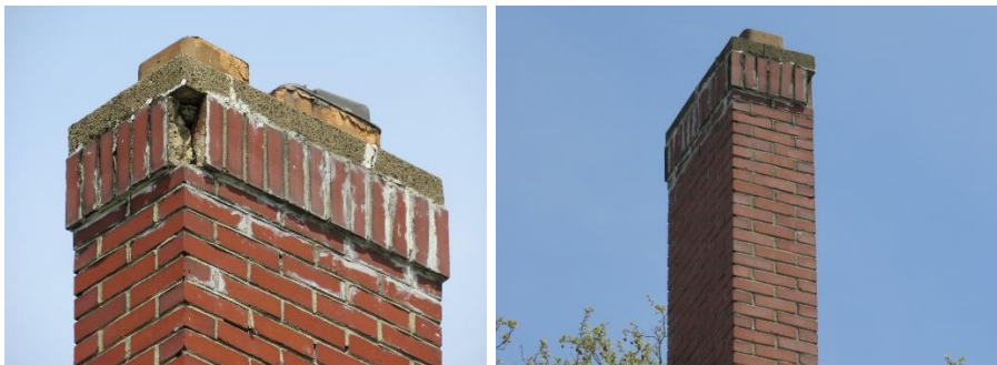
Close-up views of the central chimney
