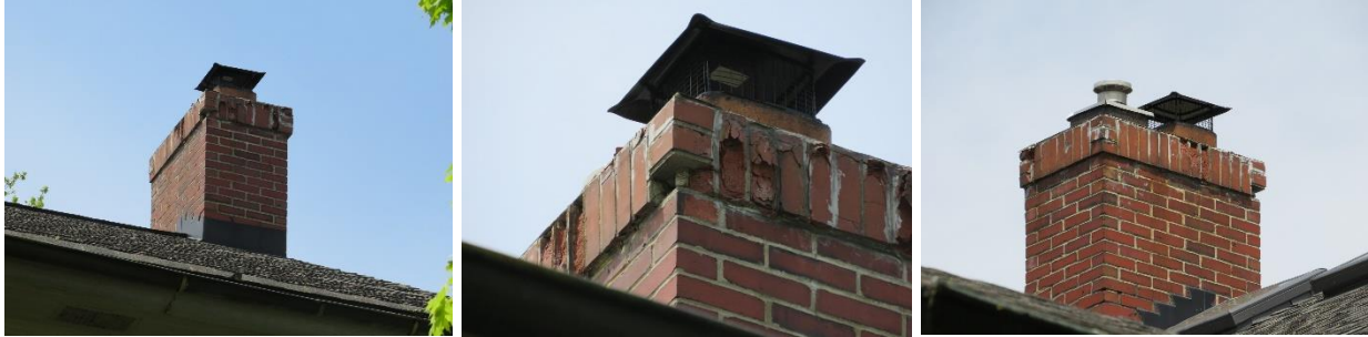
Close-up views of the north chimney
