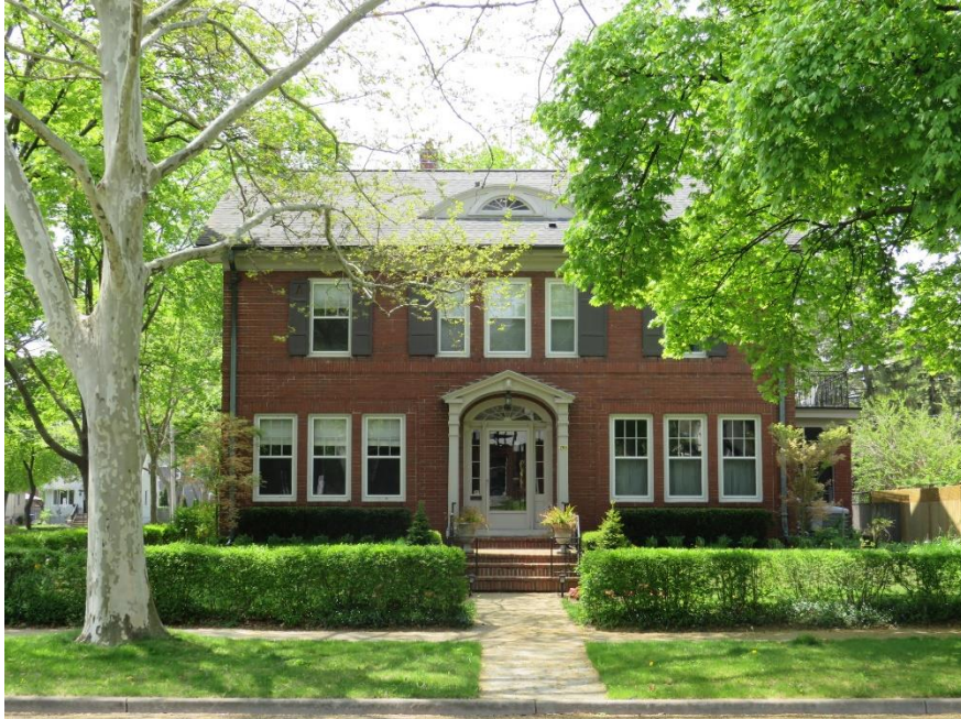
View of the front facade of 793 Devonshire Road
