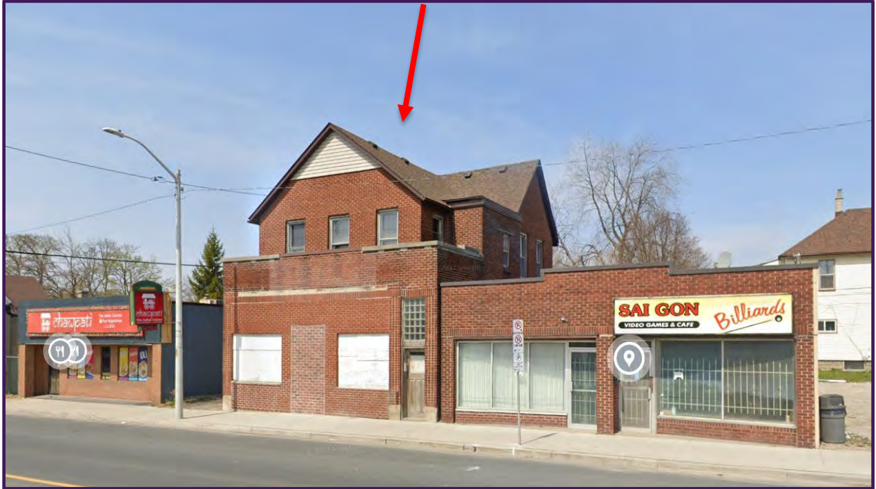
FIGURE 4: SITE PHOTO B – EAST SIDE BLDG
