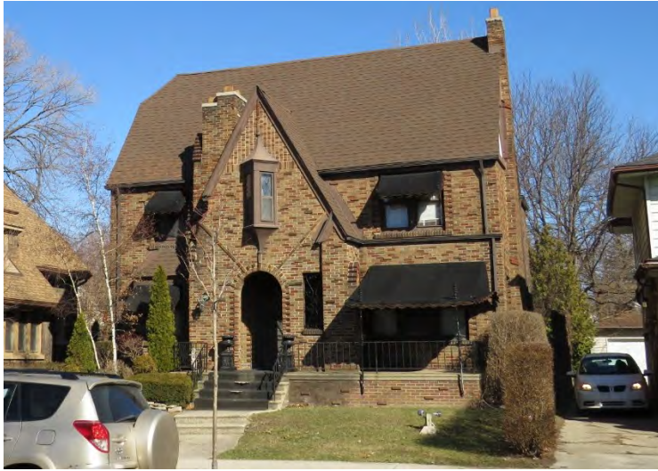
Front elevation of 436 Askin Avenue
