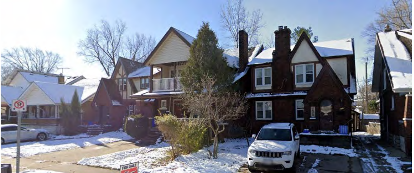
Views of the rear-abutting properties on Randolph Ave looking slightly north-west (top) and south-west (bottom).
