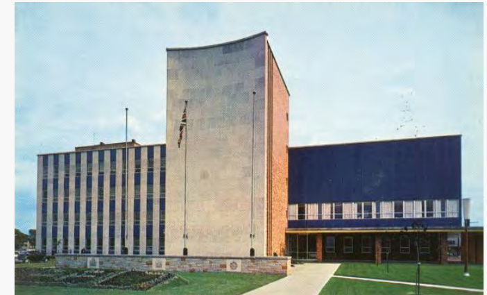
1957 City Hall. A portion of the curved wall façade has been preserved and integrated into the new concept.
