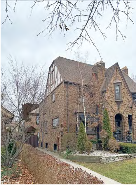
Askin Avenue-view rendering of the historic Tudor Revival style dwelling with the proposed ADU at rear
