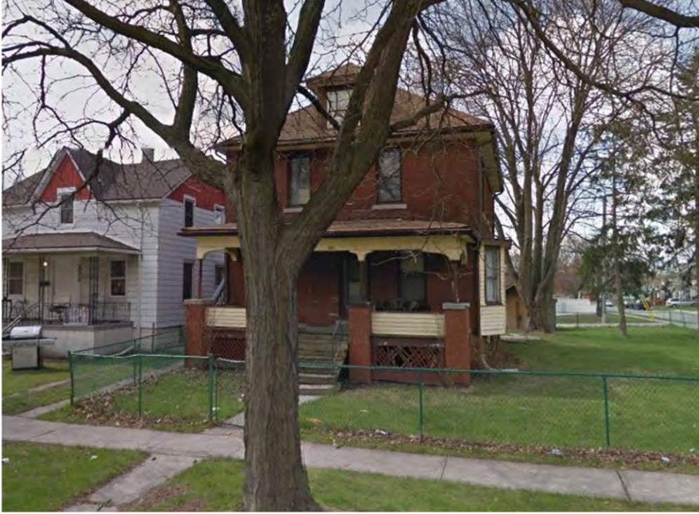
511 Brock Street Prior to Demolition
