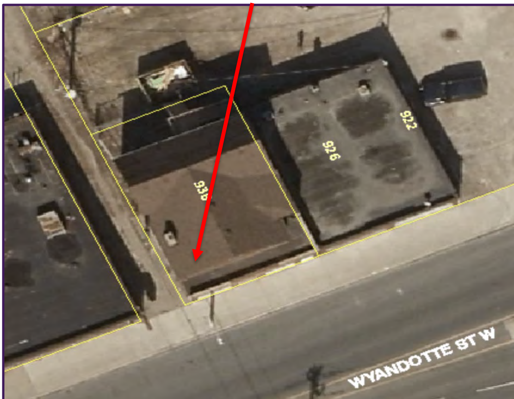
FIGURE 2: SITE AERIAL – 936 WYANDOTTE ST WEST
