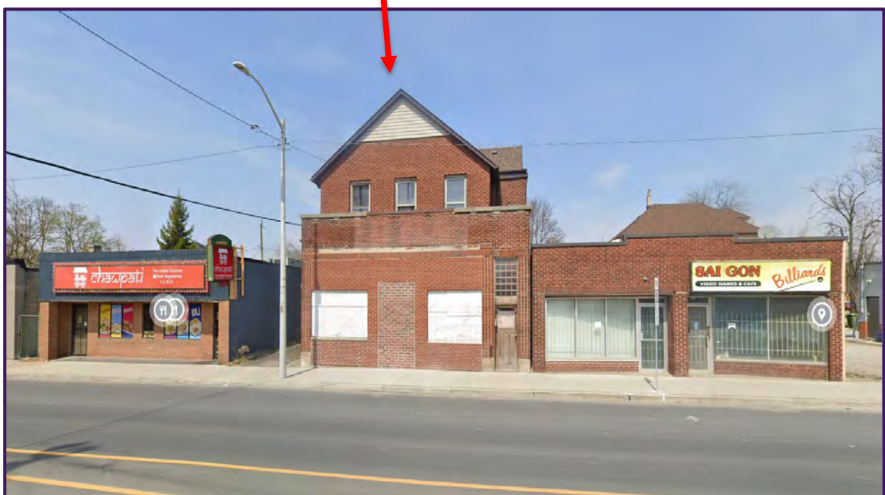
FIGURE 3: SITE PHOTO A – FRONT ELEVATIONS
