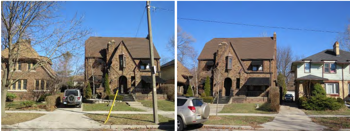
Views of the front facade of 436 Askin Avenue from Askin Avenue looking east down the left and right side yards of the property. The proposed ADU would be screened from view at these angles (photos taken in February 2023).
