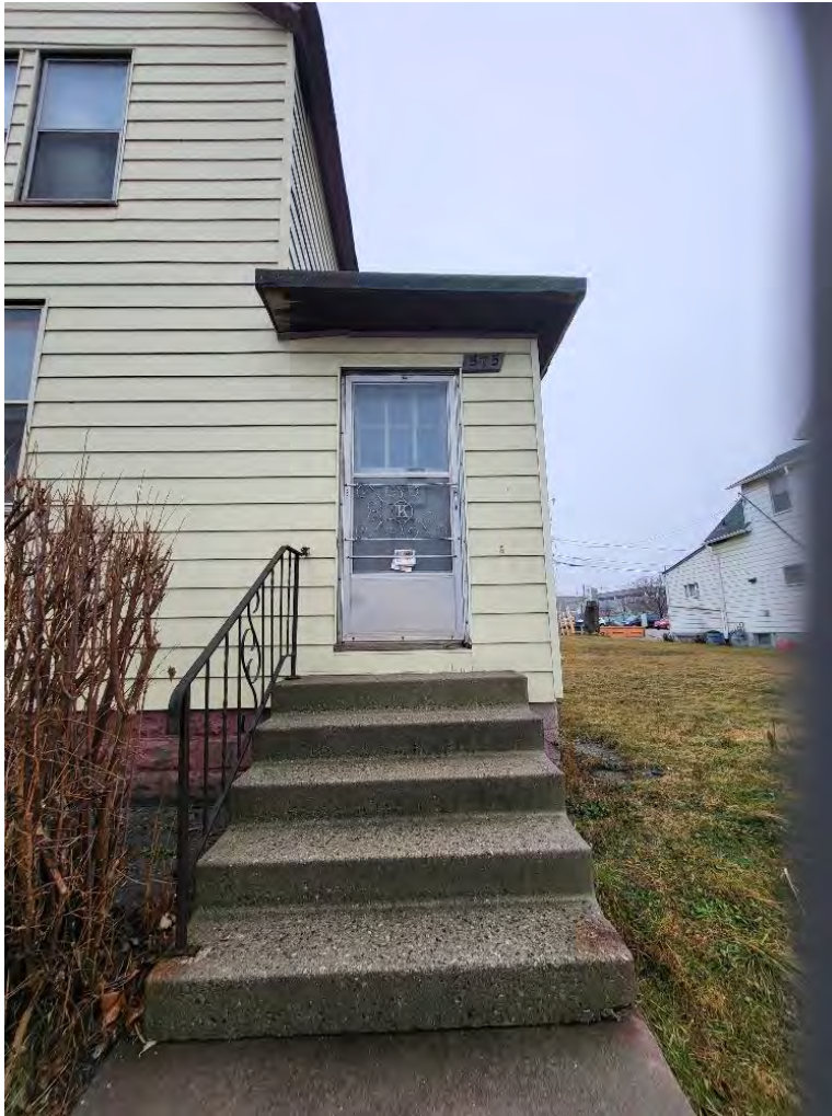
2. Front of building (North elevation).
