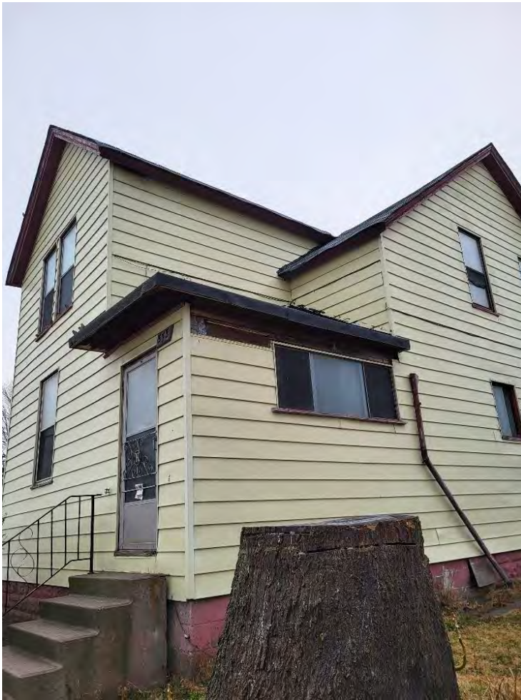
5. Side of building (West elevation).
