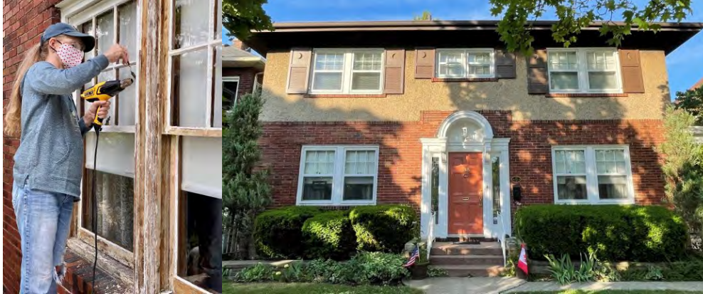
Owner conducting maintenance of painting on wood windows.
