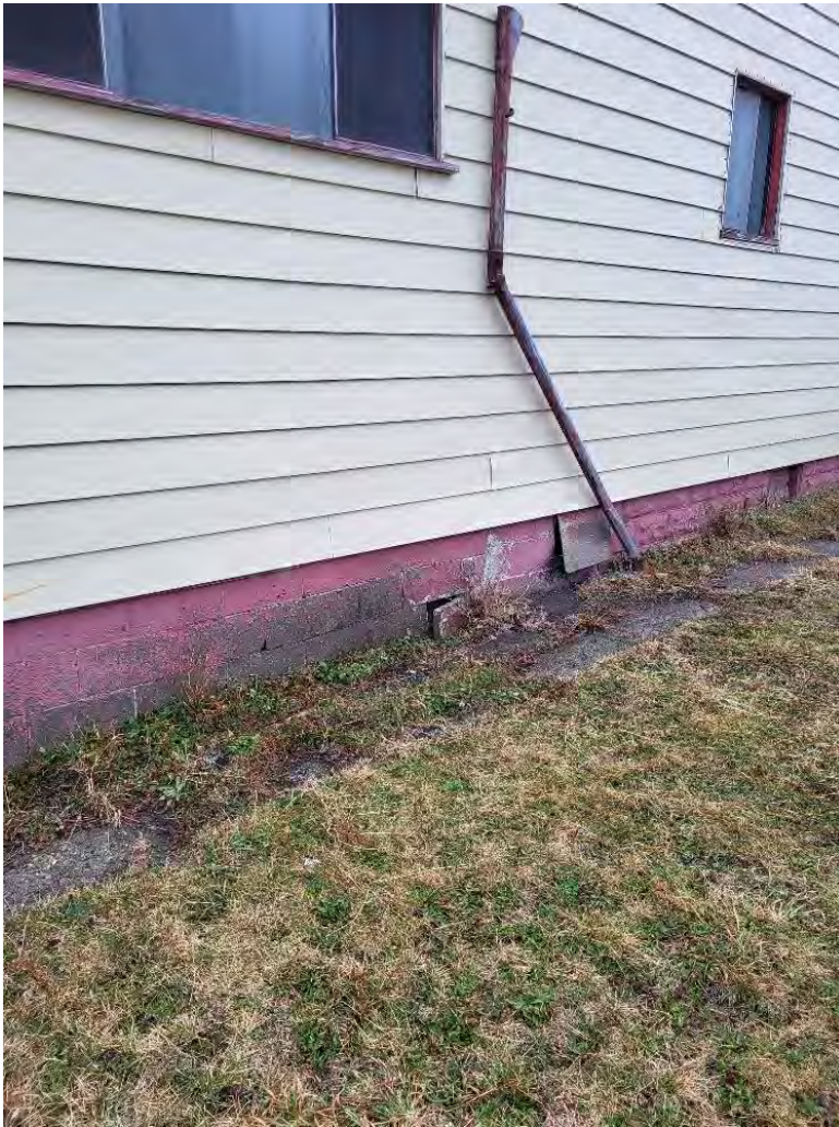
7. Side of building (West elevation).
