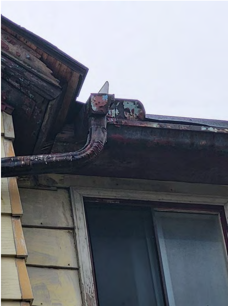
6. Roof line close up at side of building (West elevation).
