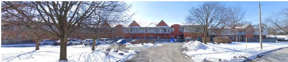
Former Ivor Chandler School (Source: Google Streetview)
