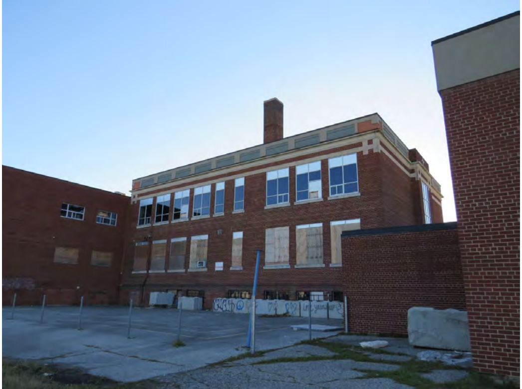
Rear of original construction
