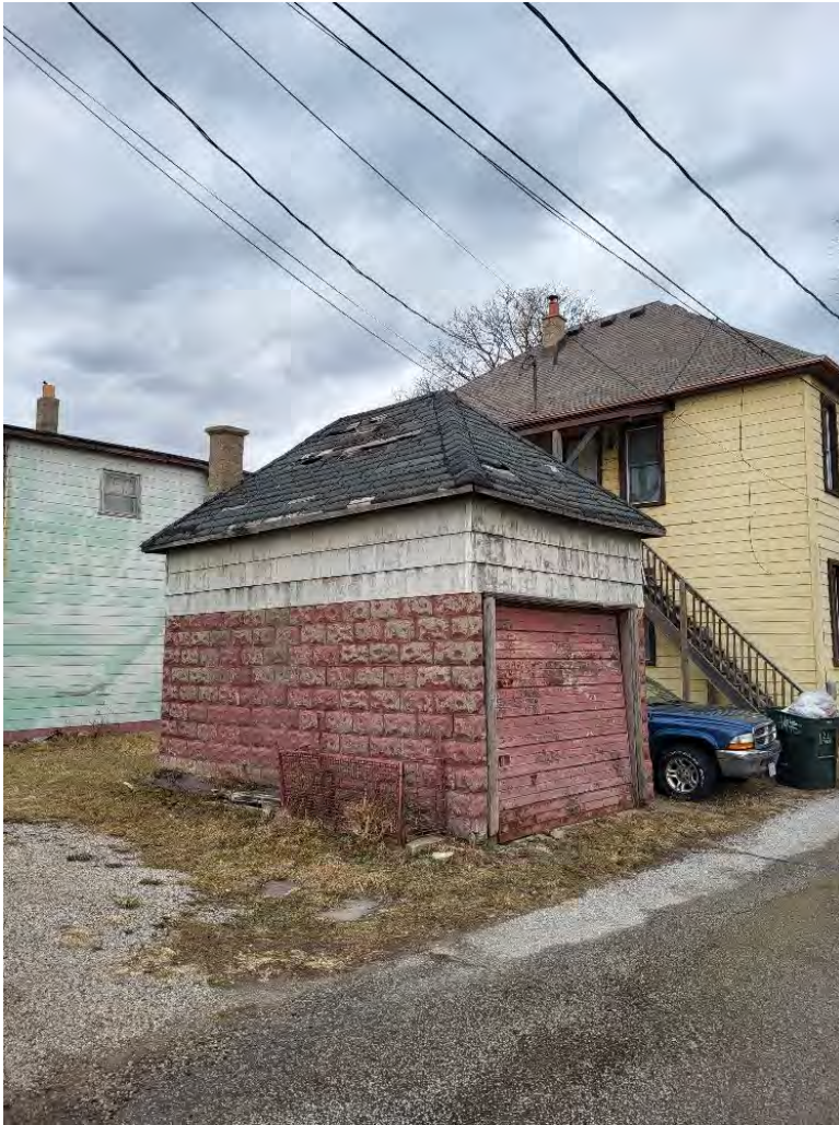
1. Rear accessory structure.
