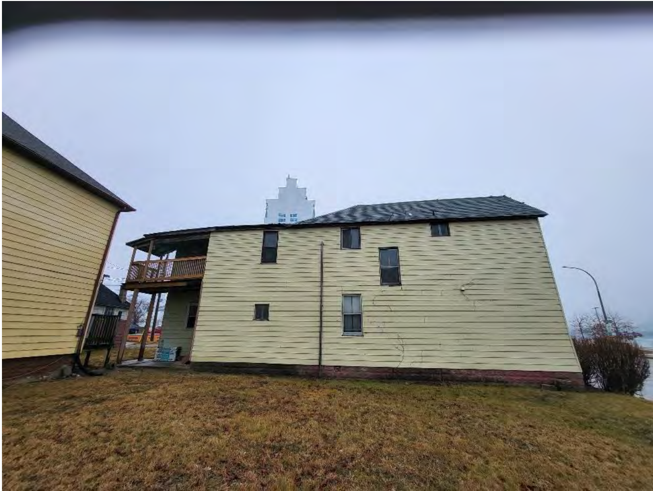
4. Side of building (East elevation).
