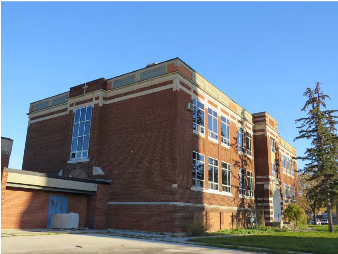
Northwest corner of property showing 1965 Gymnasium addition
