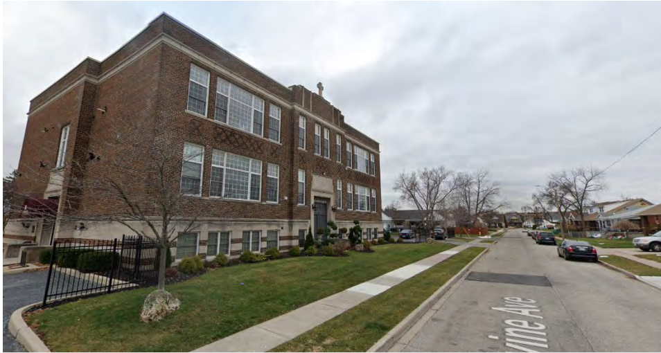
Former Ste. Genevieve School (Source: Google Streetview)
