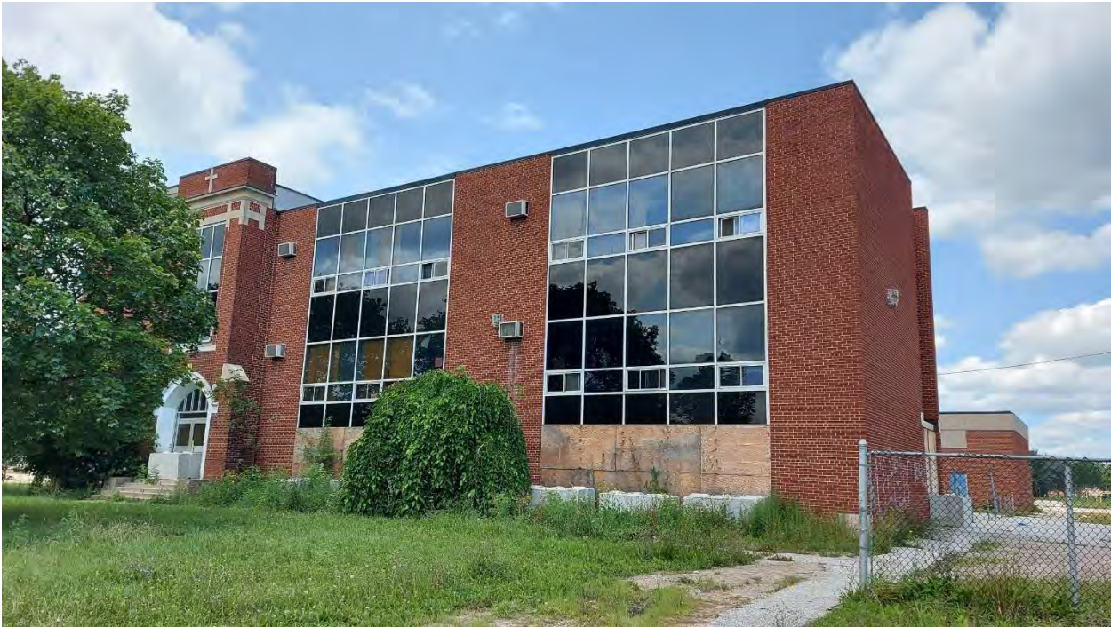
South Side elevation with 1960 addition
