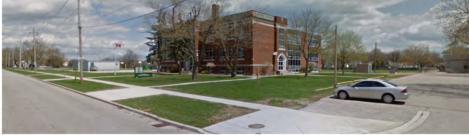
Google Streetview of property from the southwest corner of the property in May 2014.
