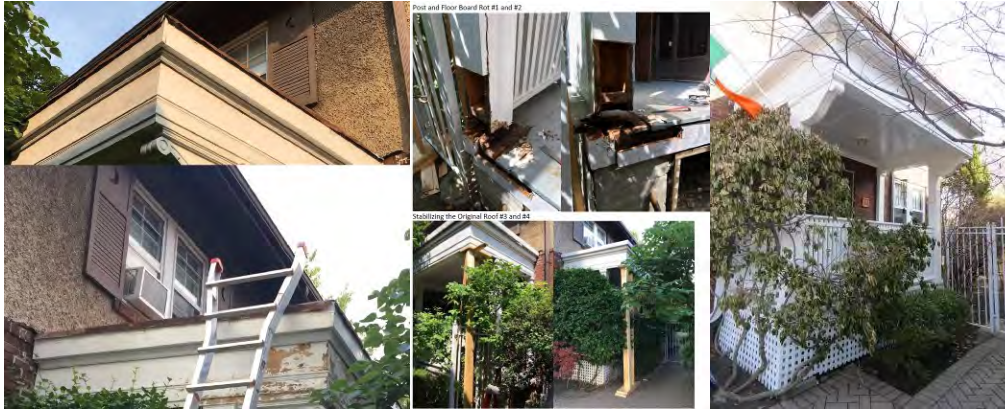
Before and after photos of the wood side porch restoration
