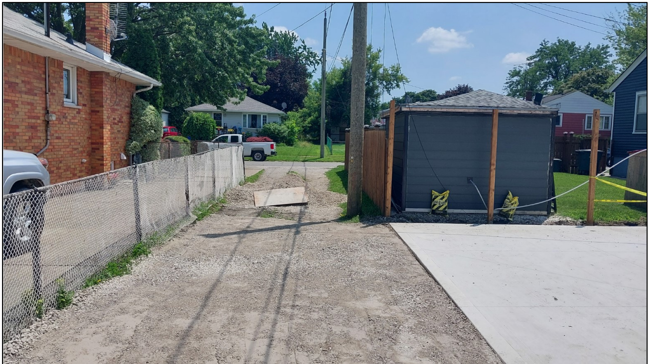
Figure 4 - Looking south from midpoint of alley (1660 Taylor Avenue on left)
