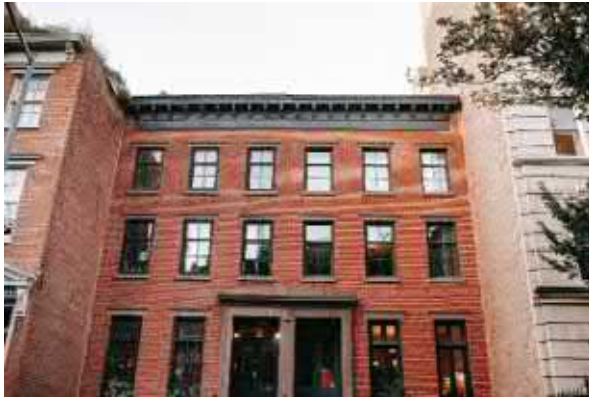
Example of architectural articulations and window fenestrations
