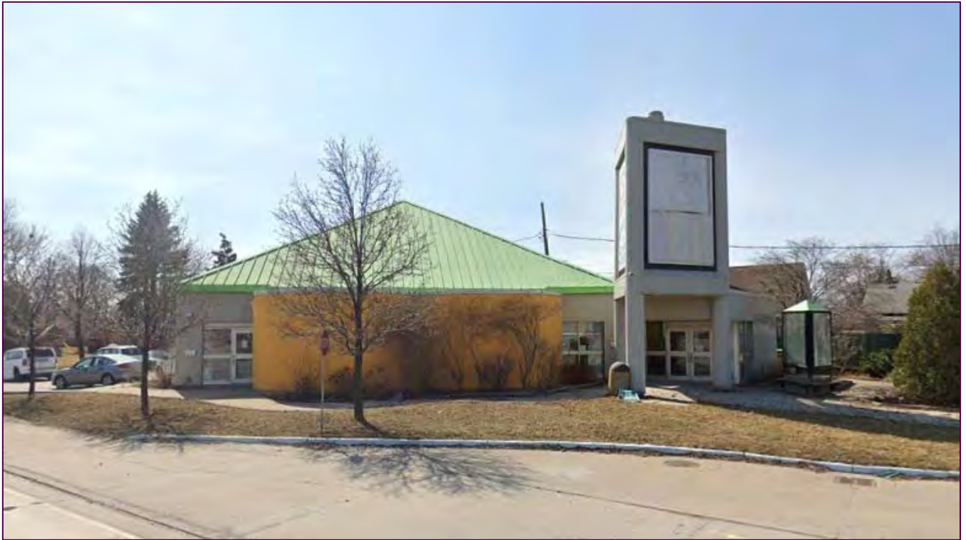
FIGURE 4 - EXISTING BUILDING (FORMER TOURIST BUREAU)
