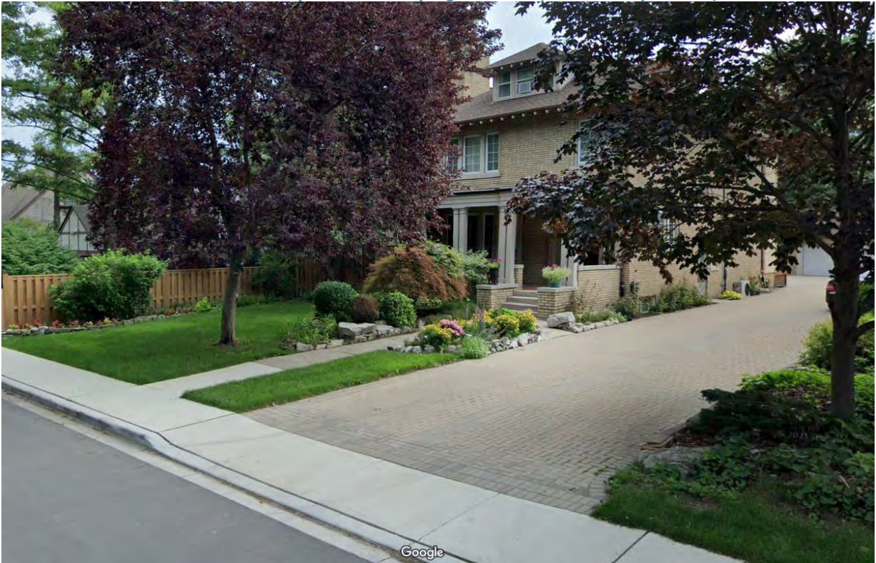
Figure 20 - Example of Landscaping Features (166 Randolph Place)
