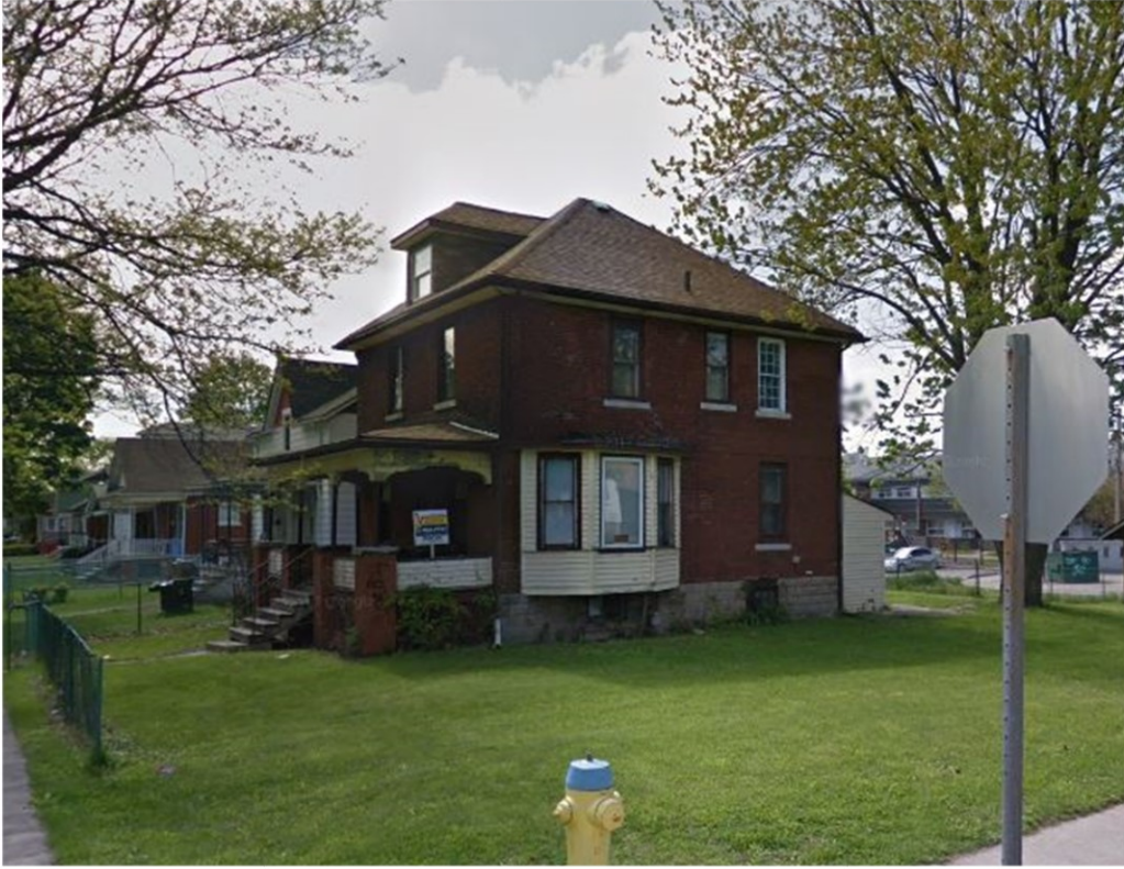
511 Brock Street Prior to Demolition
