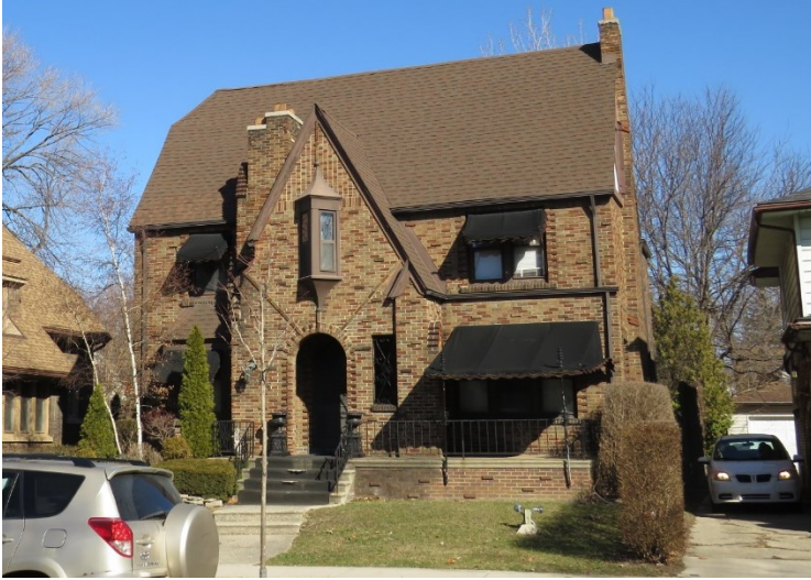
Front elevation of 436 Askin Avenue
