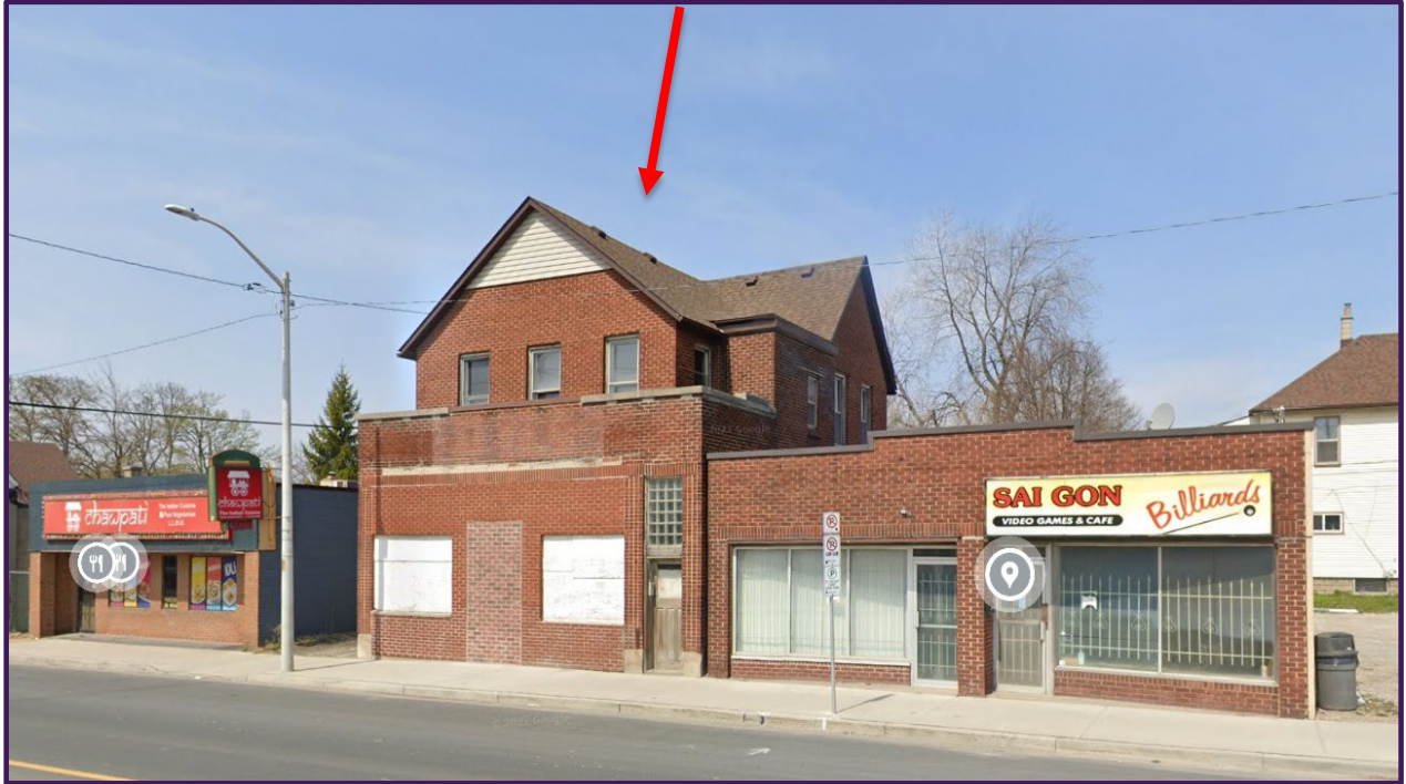
FIGURE 4: SITE PHOTO B – EAST SIDE BLDG
