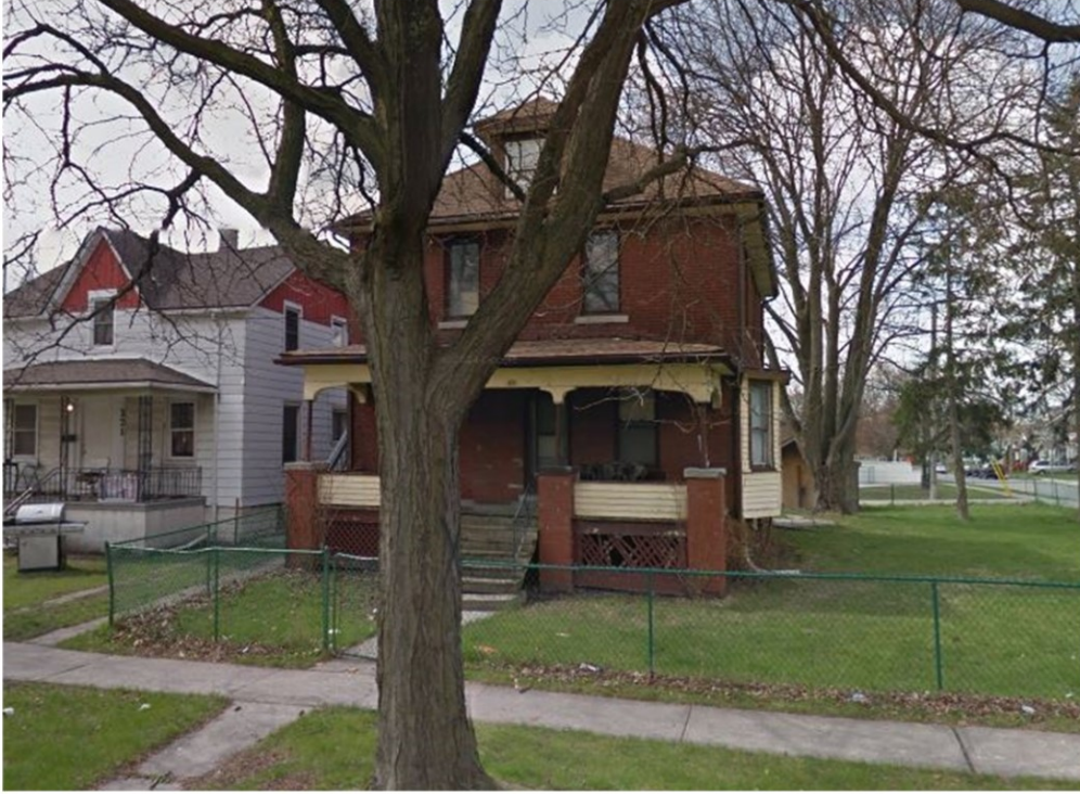
511 Brock Street Prior to Demolition
