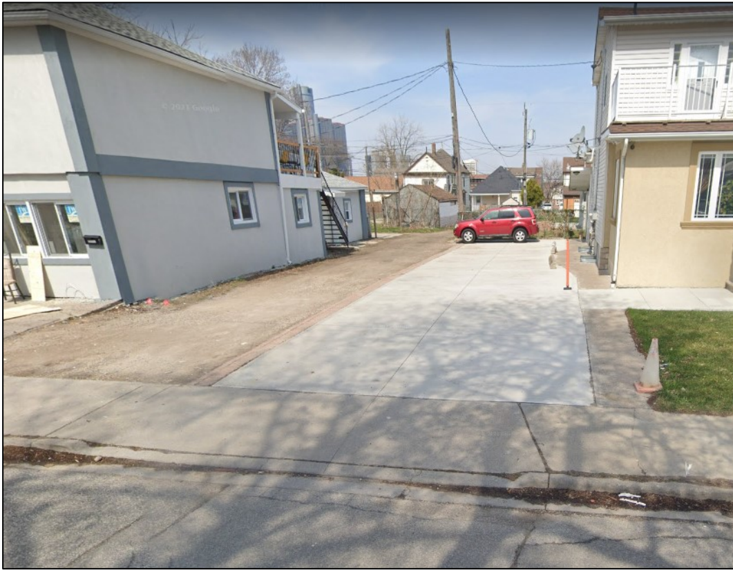
Figure 15 - Looking north towards City owned lane from University Avenue East (April 2021 Google Street View); 836 University Avenue East to right
