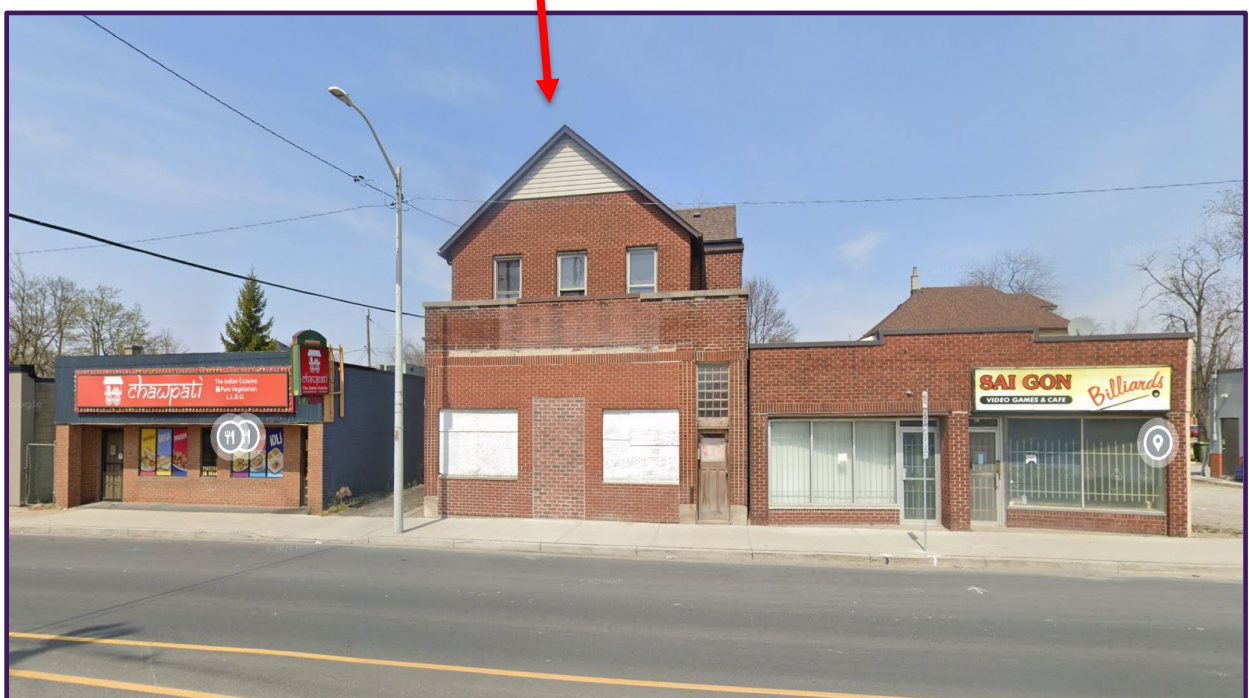
FIGURE 3: SITE PHOTO A – FRONT ELEVATIONS
