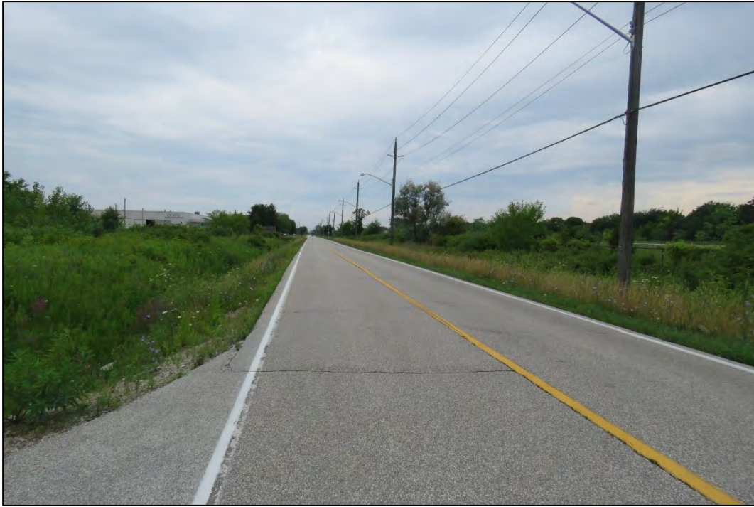
Figure 1 - E. C. Row Avenue East looking west from driveway at 9455 Anchor Drive
