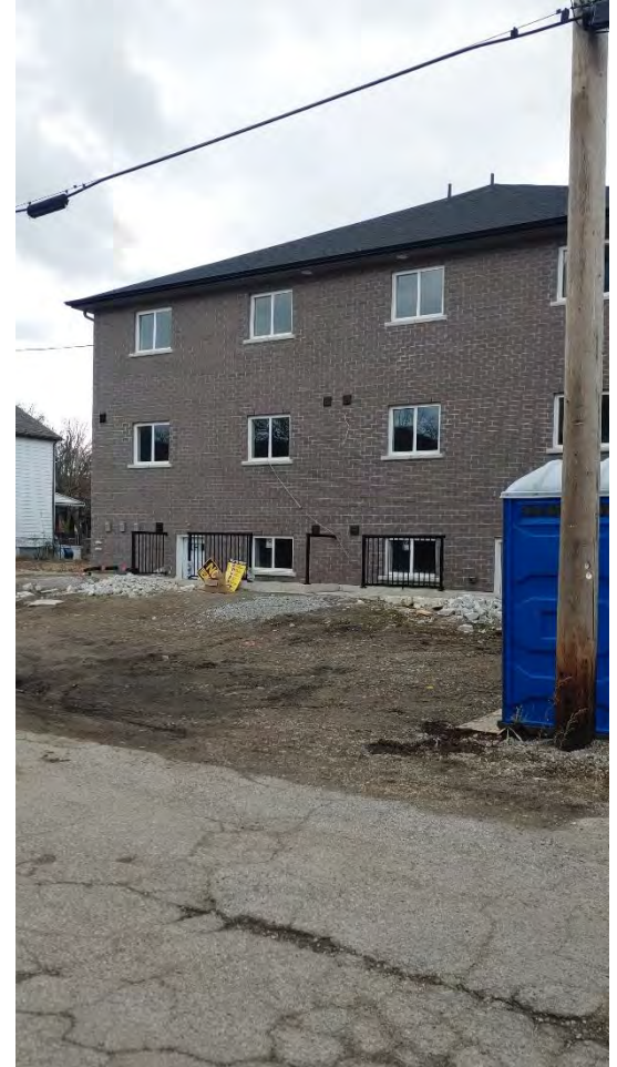
View of subject 4-plex from abutting rear alley.
