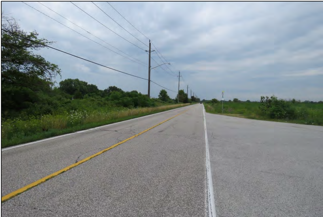
Figure 2 - E. C. Row Avenue East looking east from driveway at 9455 Anchor Drive
