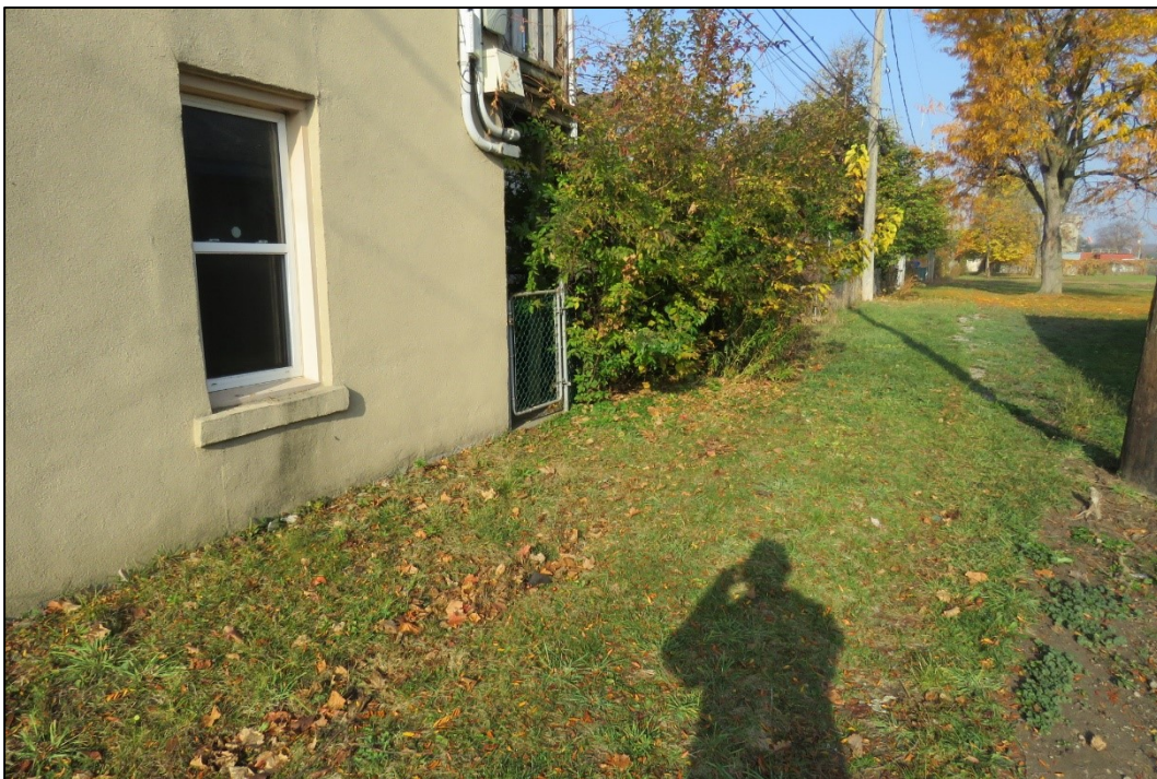
Figure 12 - North/south alley looking north (1636 Seneca Street on left)
