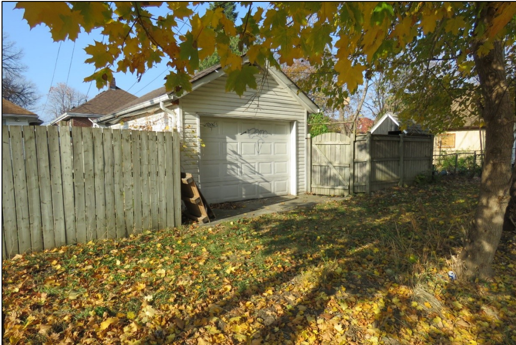
Figure 18 - North/south alley looking north towards rear detached garage at 1638 Lincoln Road
