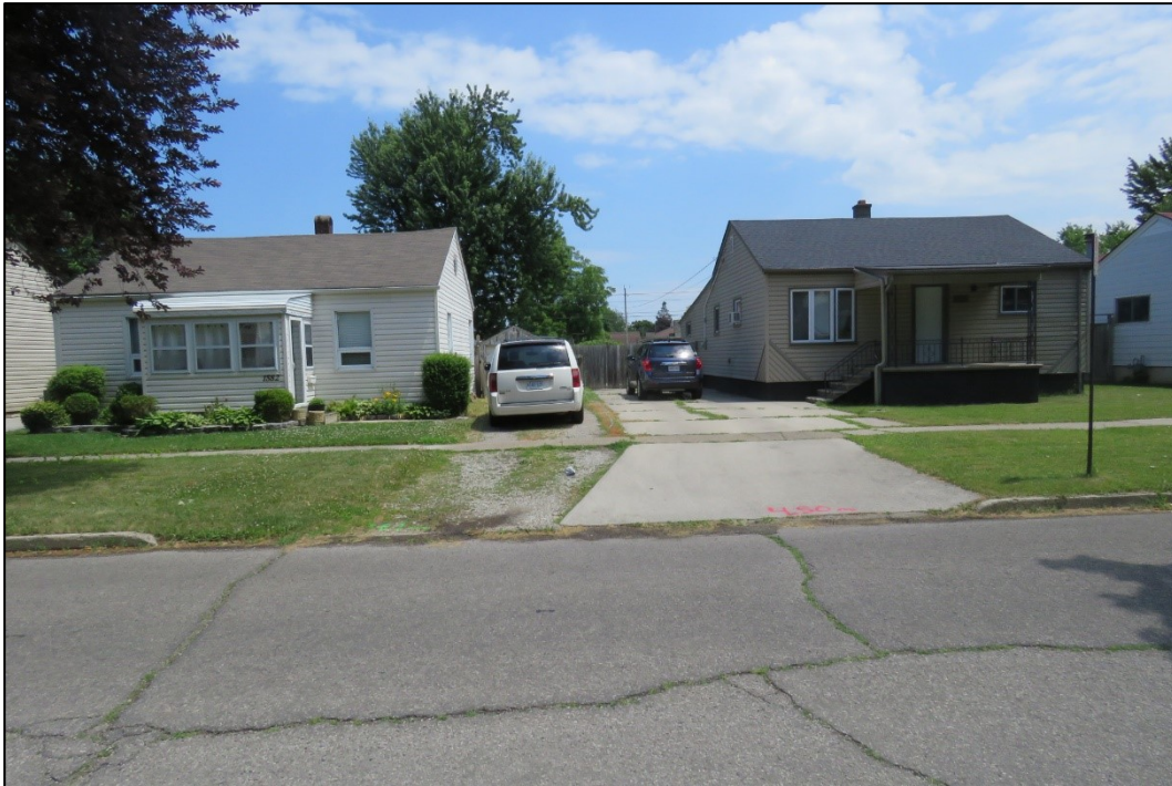
Figure 1 - Looking east towards alley from Aubin Road (1590 Aubin Road on right)
