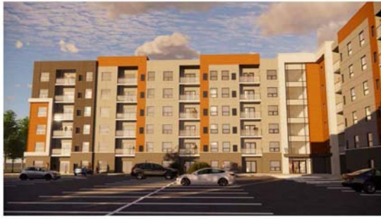
REAR - NORTH - FRONT ENTRANCE
