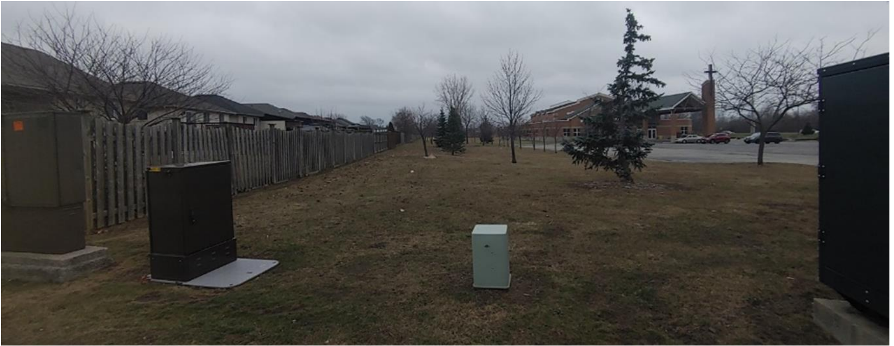
Existing wooden fence between the 2400 Banwell Rd) and the SUDs fronting on Tranquility Ave.
