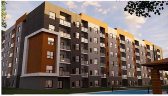
REAR - SOUTH EAST CORNER
