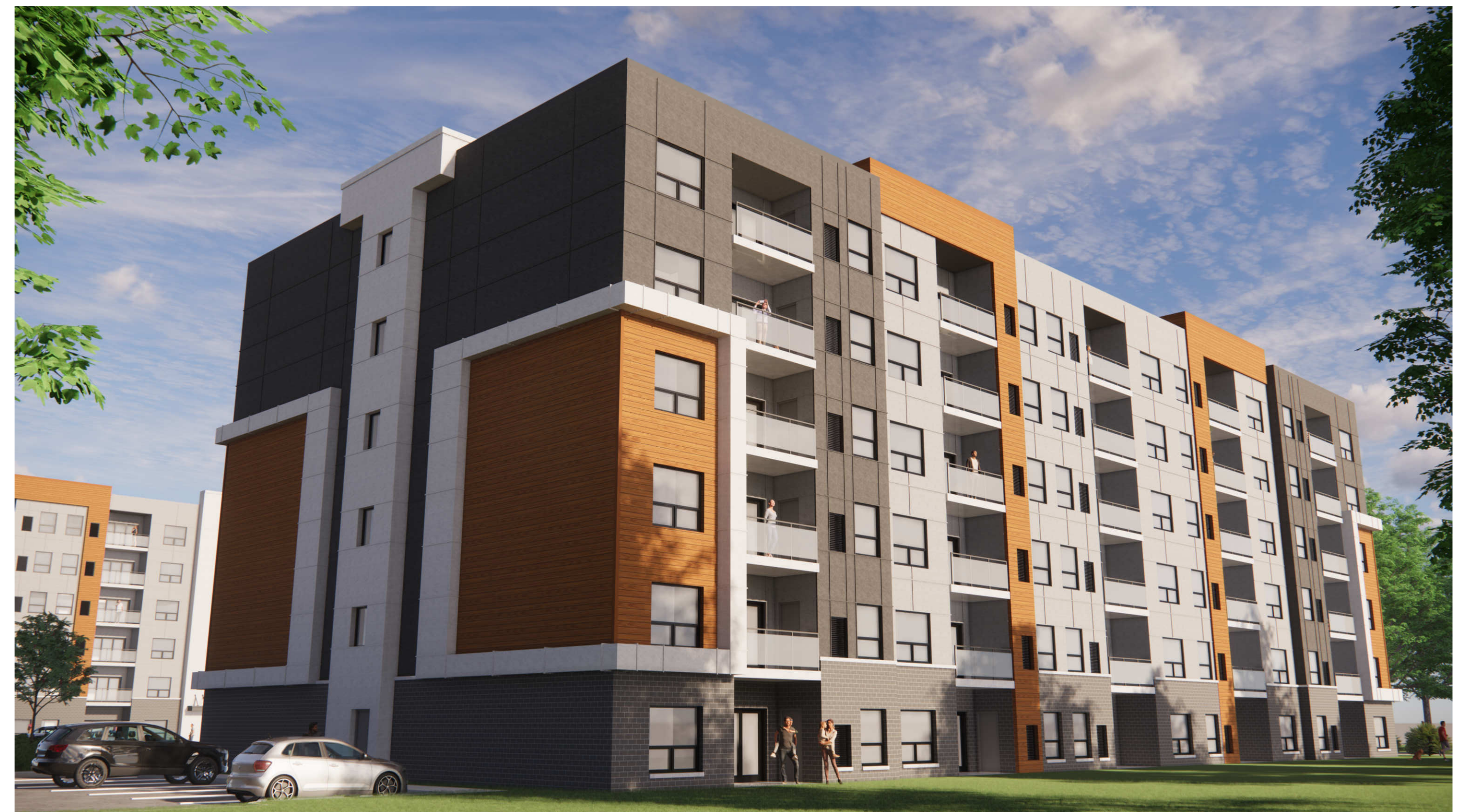
REAR - SOUTH EAST CORNER
