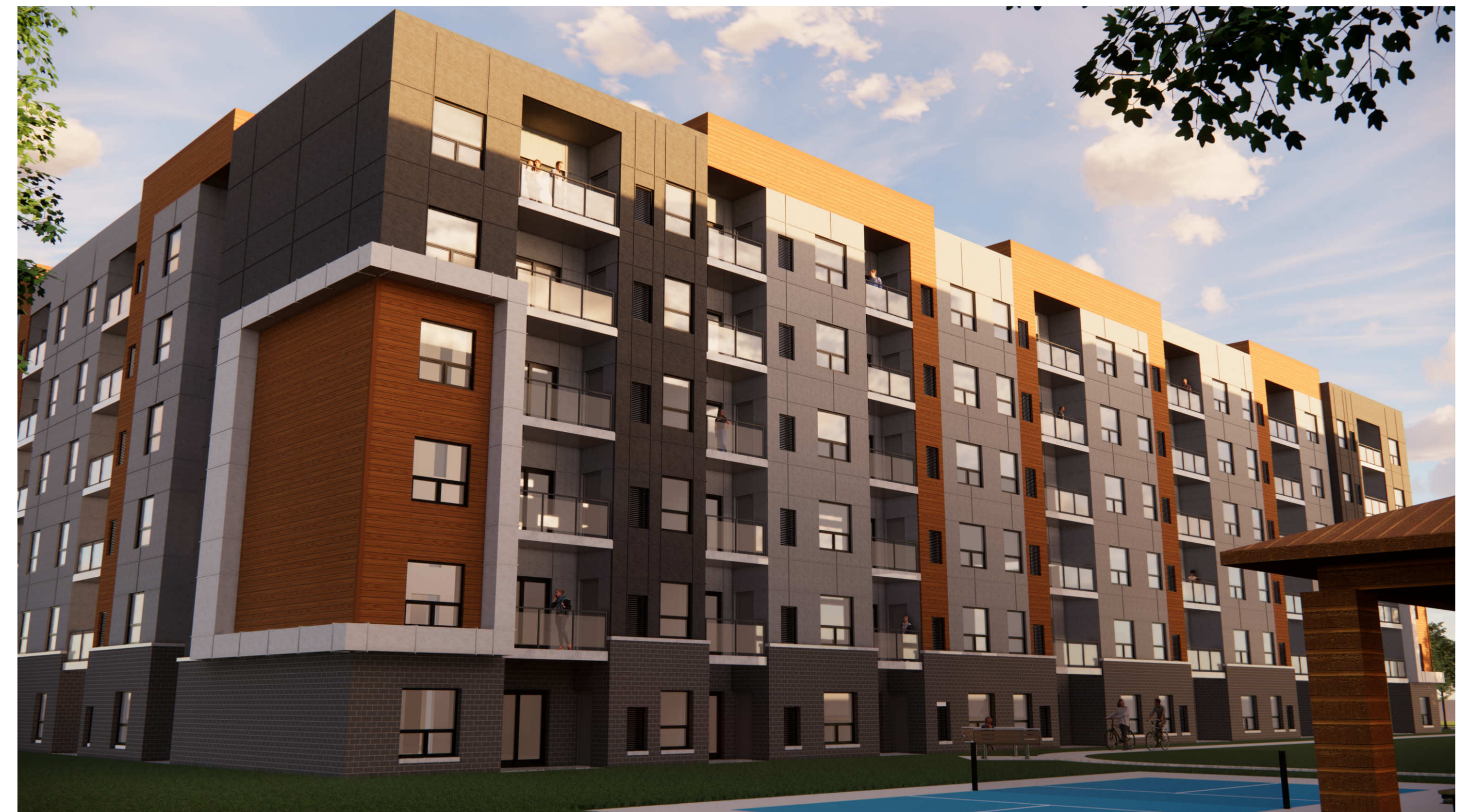
REAR - SOUTH EAST CORNER
