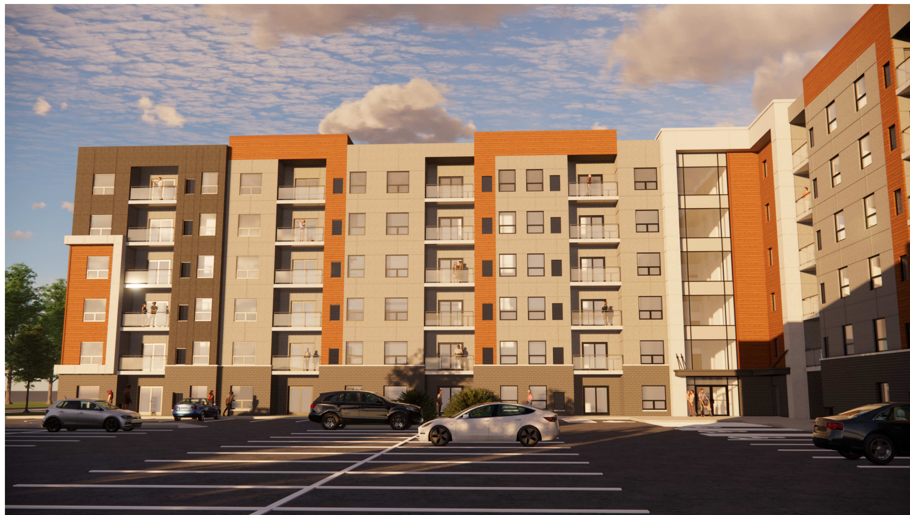
REAR - NORTH - FRONT ENTRANCE
