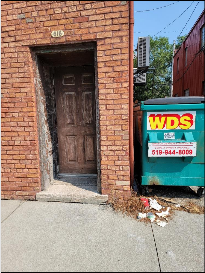
Figure 6 - Looking east towards alley from Chilver Road (616 Chilver Road on left)
