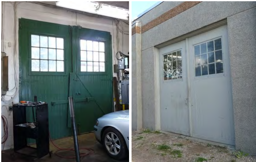
Photographs of the wood doors interior and exterior, taken September 2016
