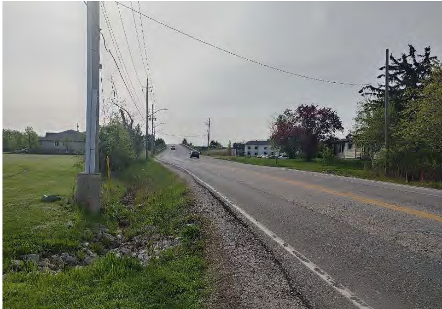
VIEW OF NORTH TALBOT, LOOKING EAST AT OLD WEST AVENUE, SHOWING FRONTAGE OF 1085 and 1255 NORTH TALBOT RD
