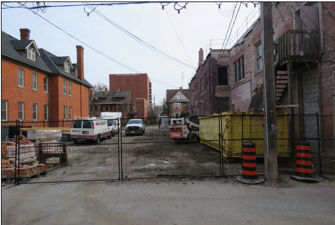
Figure 8 - Rear of 1958-1998 Wyandotte Street East, looking east from subject alley
