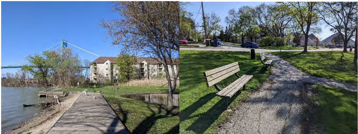
Photographs of McKee Park in May 2022 showing current state of the boardwalk, drainage issues, pathways, and benches.
