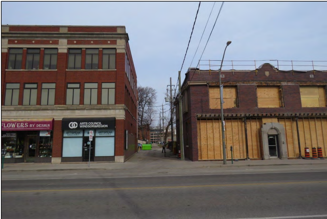
Figure 1 - Looking north towards subject alley from Wyandotte Street East
