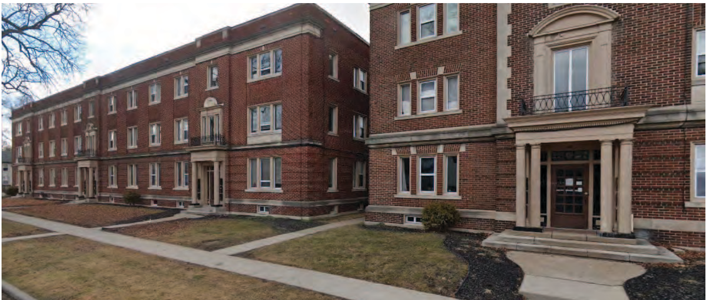
Three storey apartment buildings on Argyle Street in the Walkerville neighbourhood.
