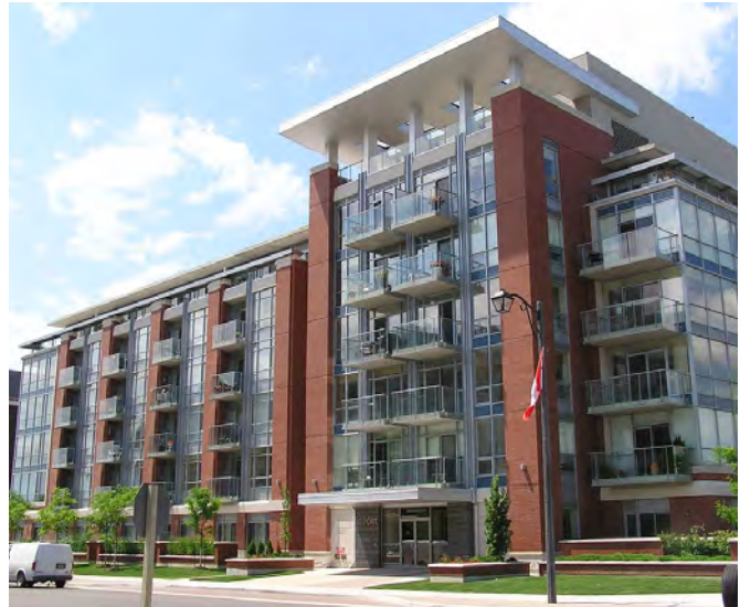
Example of a 6 storey residential building.
