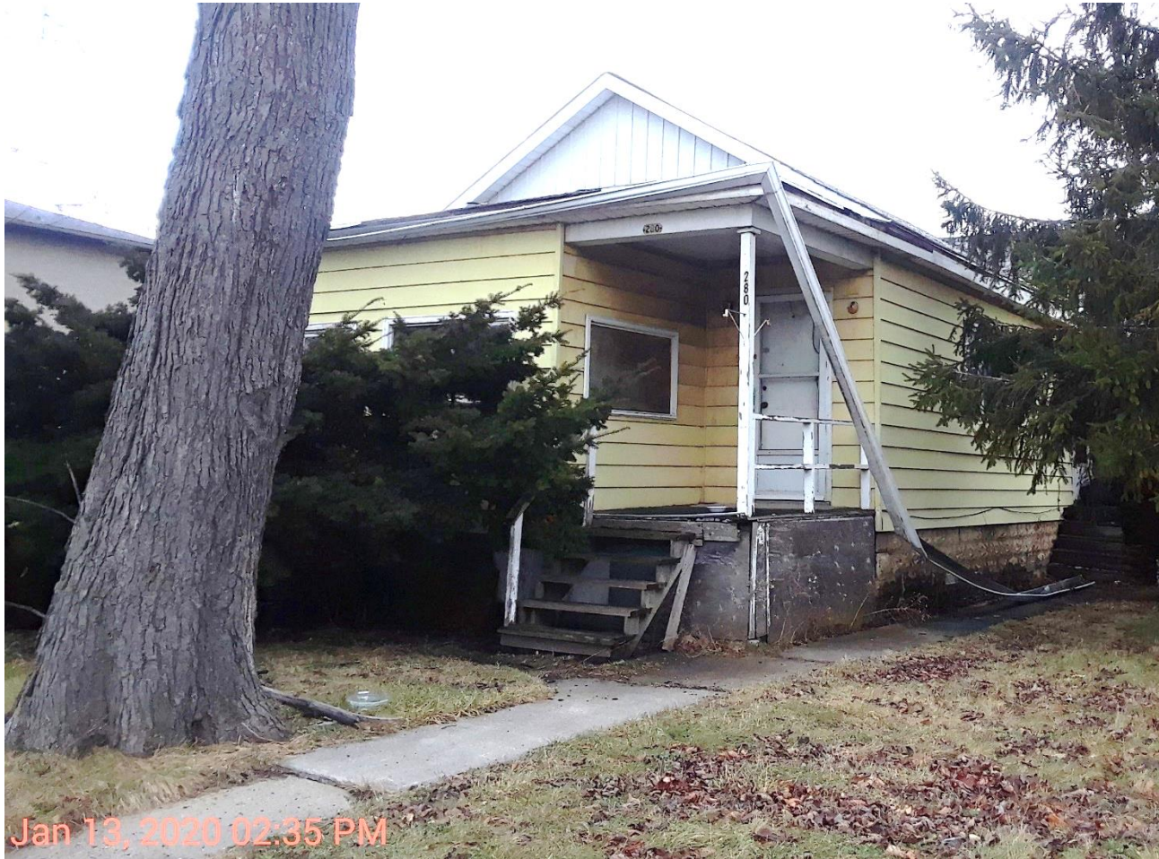
Front of building (West elevation)
