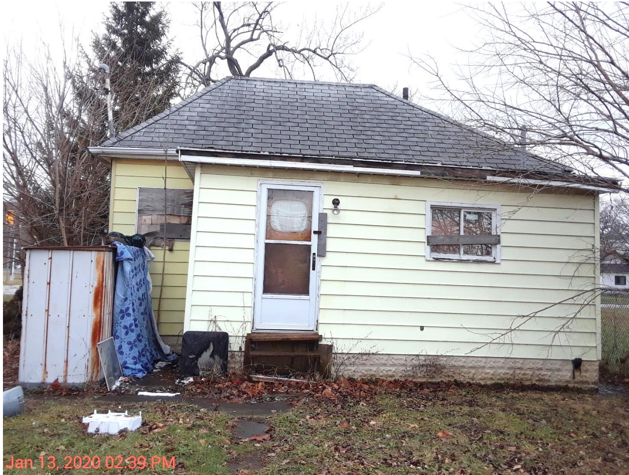
Rear of building (East elevation)
