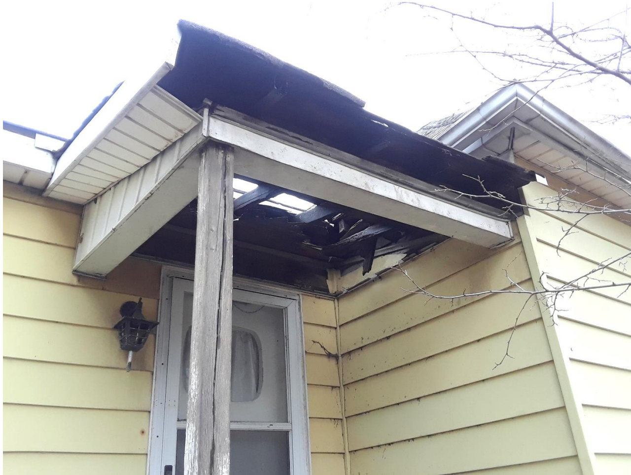
Side of building (South elevation)
