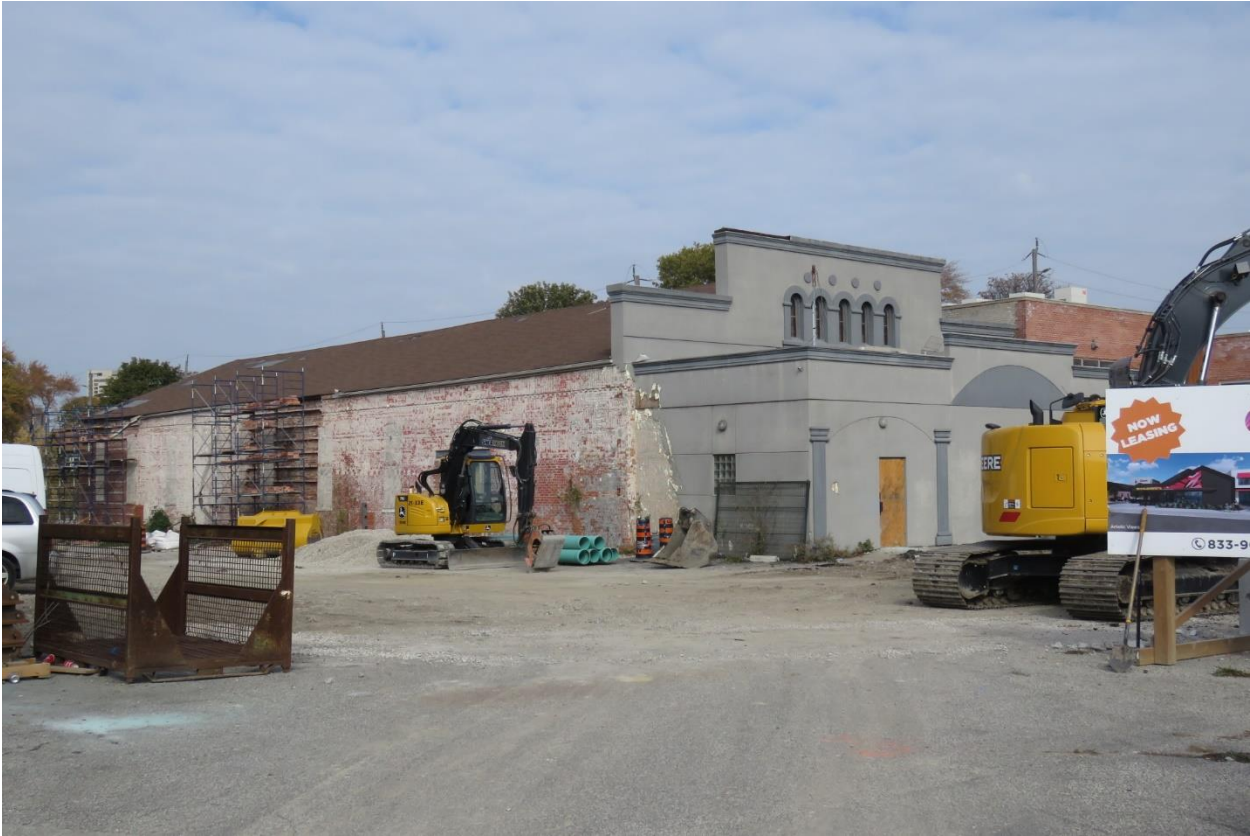
Front (south) and side (west) facades
