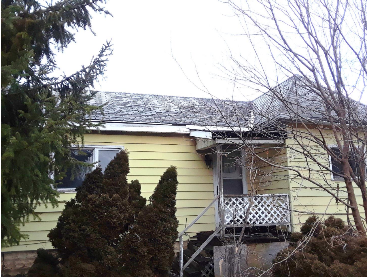
Side of building (South elevation)
