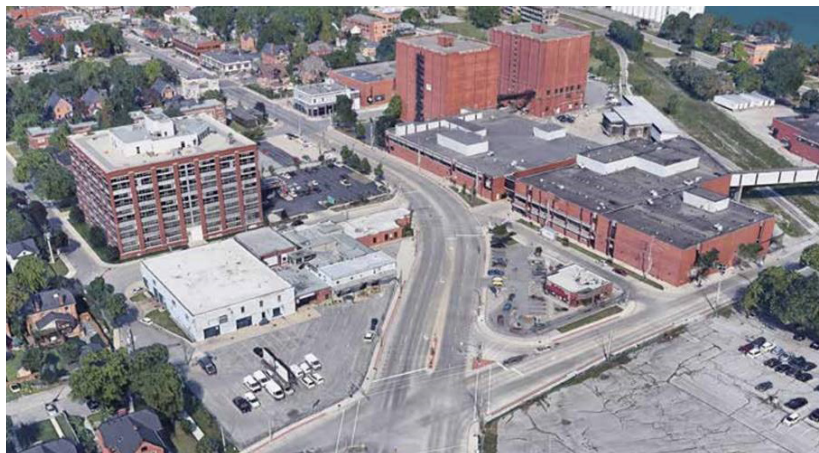
Figure 94. Bird's Eye View - Existing Condition
