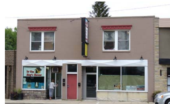
Figure 131. Original brick has been painted over, and non-traditional building materials have been added on top
