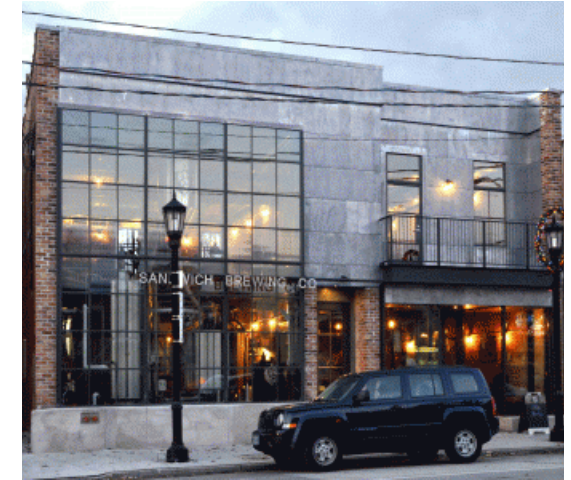
Figure 57. 3236 Sandwich Street at completion
