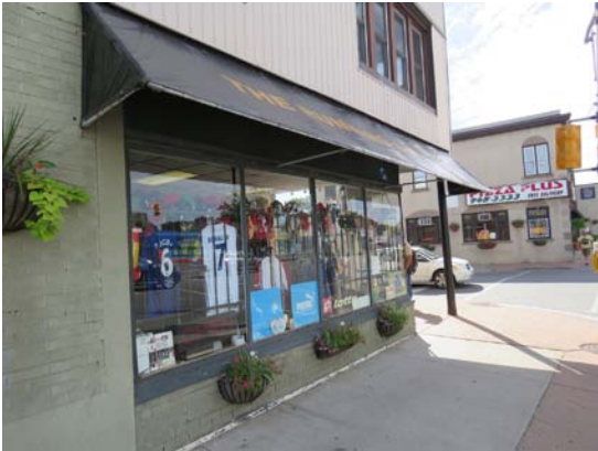
Figure 117. Bars and merchandise covering the windows impact the “indoor/outdoor” relationship with the street. Security bars give the impression that the area is unsafe
