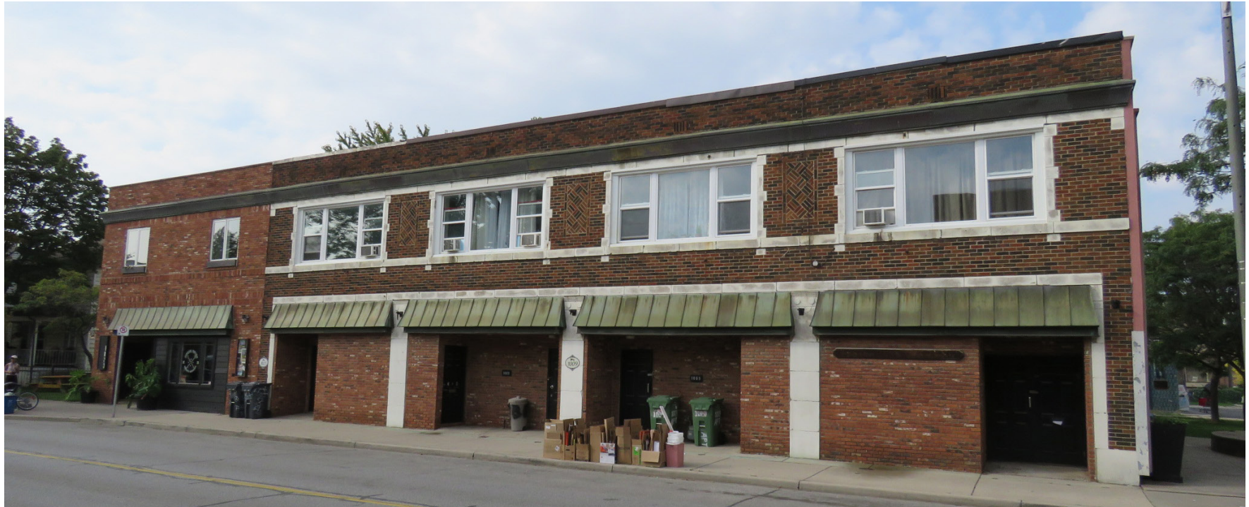
Figure 100. A building facade on the west side of Drouillard Road with original storefront windows and doors bricked in, eliminating the connection with the street
