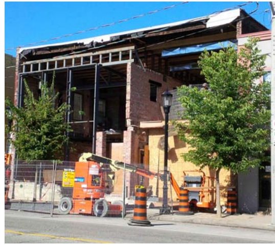
Figure 56. 3236 Sandwich Street during renovations
