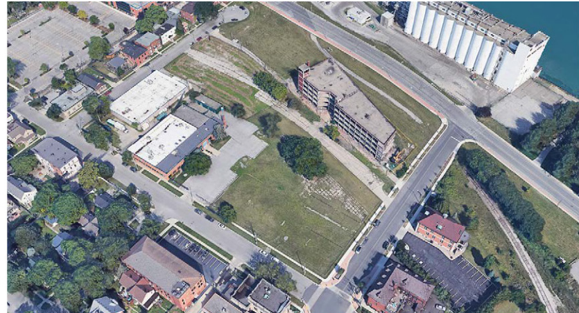
Figure 92. Bird's Eye View - Existing Condition
