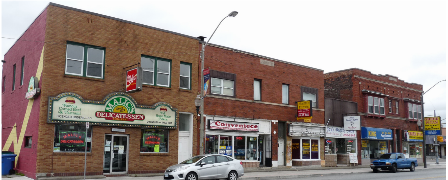
Figure 41. All store fronts are unique and are clearly distinctive through building material and architectural features
