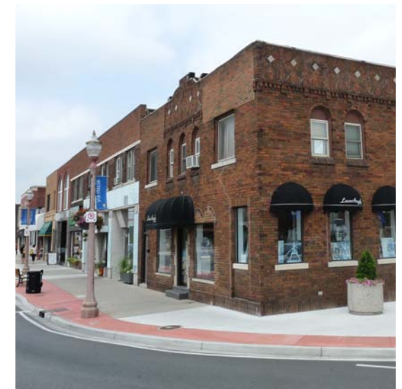
Figure 20. Erie Street and Parent Avenue, Windsor
