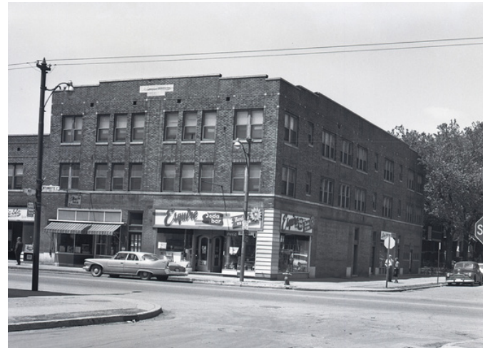
Figure 67. Leatherdale Block located at 1380-1394 Wyandotte Street East (1960)
