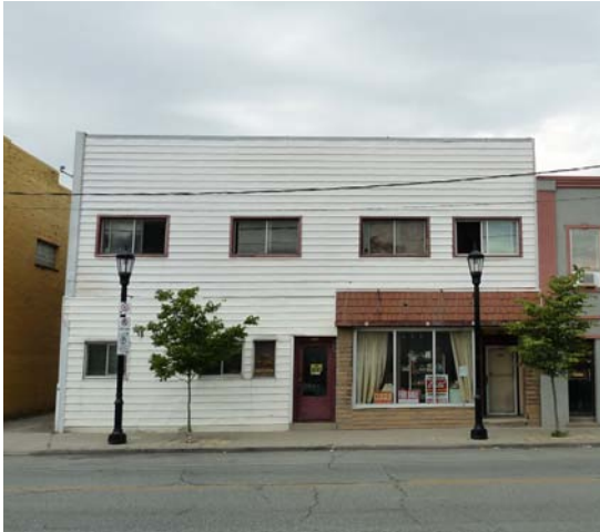
Figure 55. 3236 Sandwich Street before renovations
