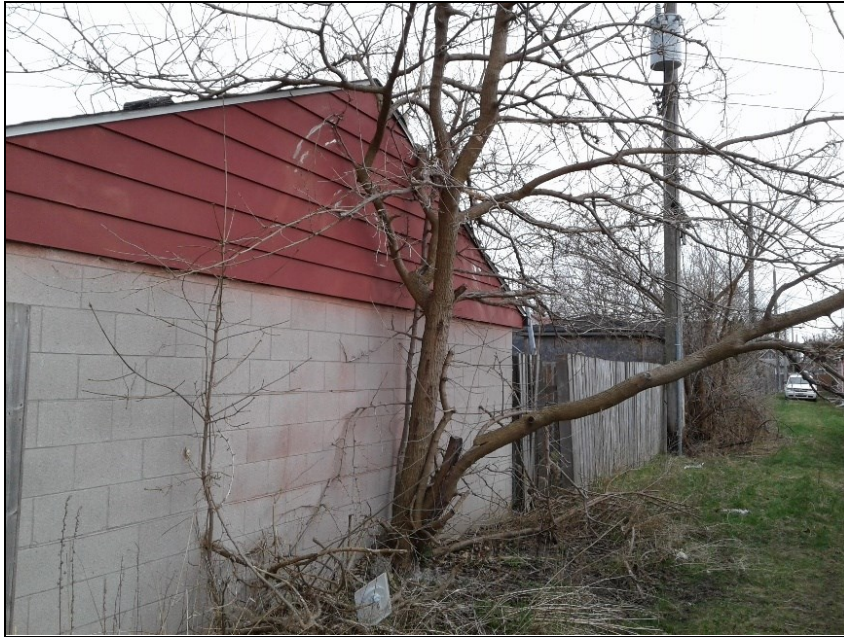
Figure 2 - Looking east from alley towards west wall of detached garage (2019)
