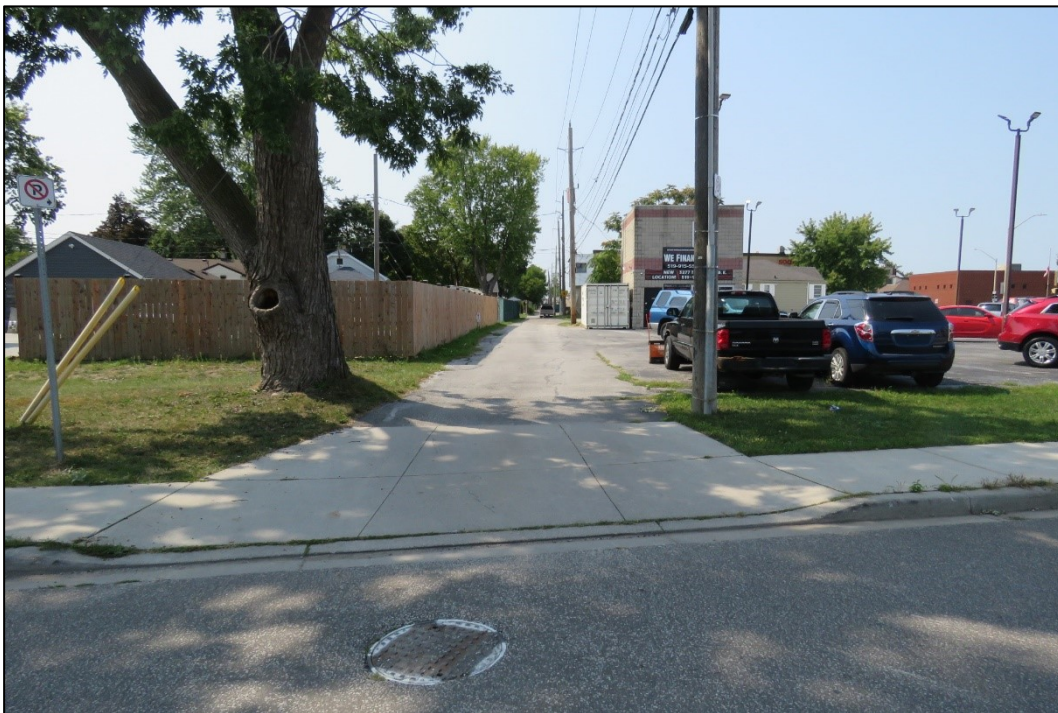
Figure 2 - Looking west towards portion of alley requested for closure from Meldrum Road
