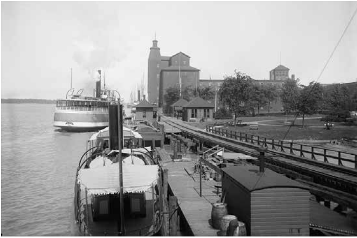
Image 1M: Ferry dock at the foot of Devonshire St. Image source: City of Windsor
