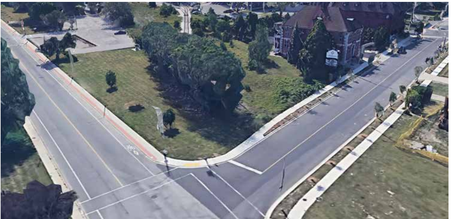
Bird's Eye View - Existing Condition
