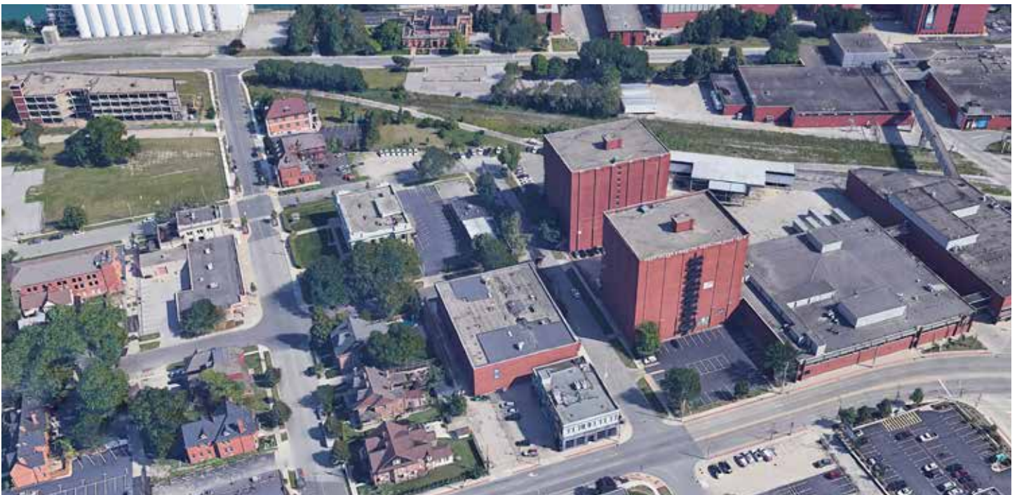
Bird's Eye View - Existing Condition
