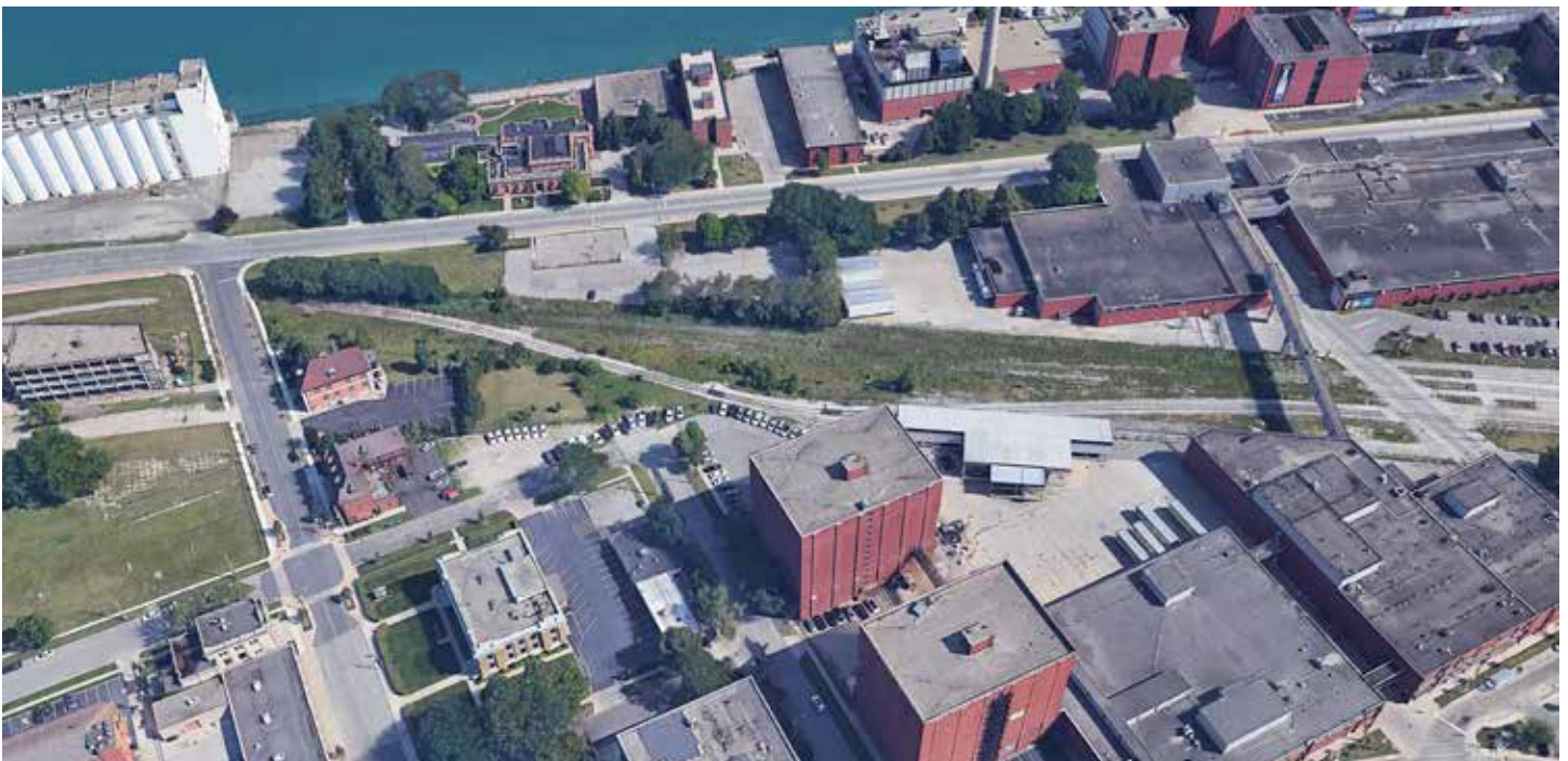
Bird's Eye View - Existing Condition
