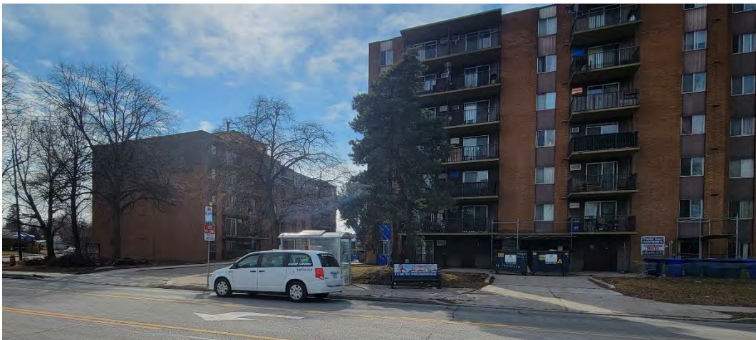
Figure 25 Example of a Bus Stop Between Access Driveways
