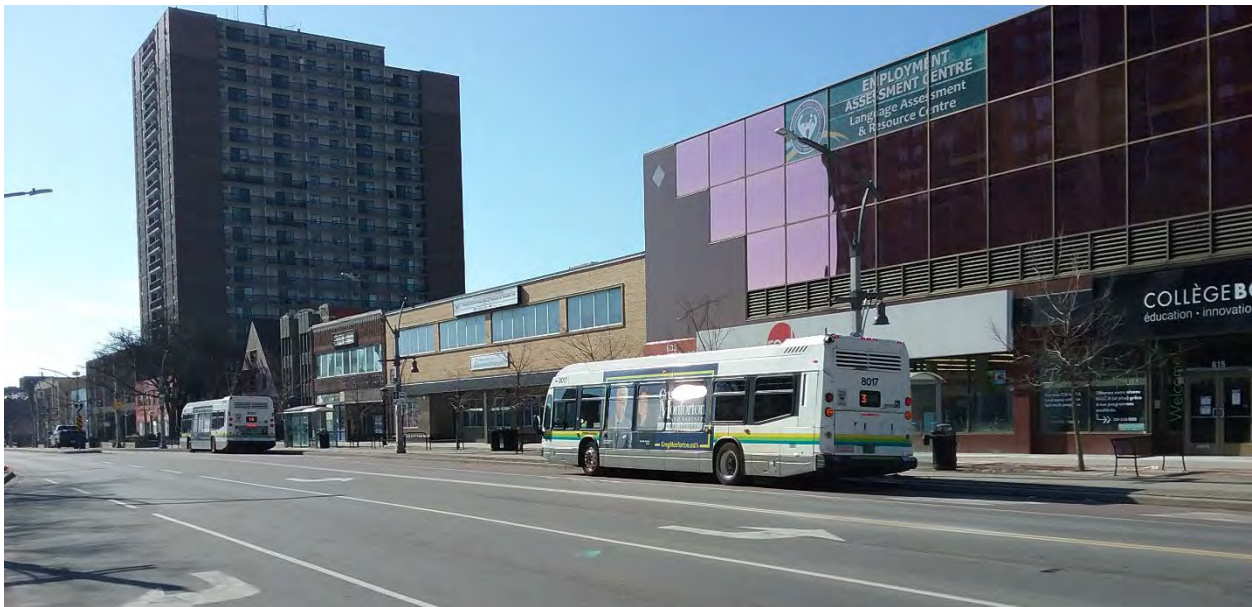
Figure 68 Transit Windsor On-Street Terminal at Ouellette and Wyandotte
