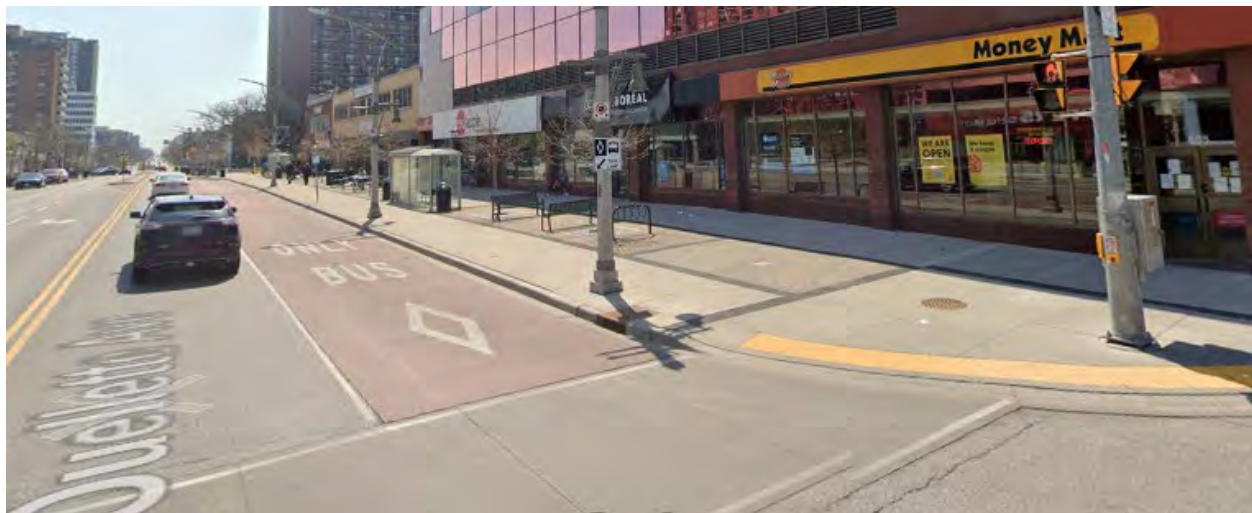
Figure 45 Example of an On-Street Bus Bay with Red Concrete
