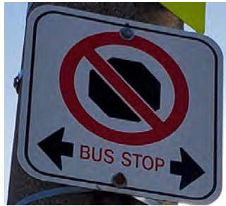
Figure 110 Example of a "No Stopping" Sign
