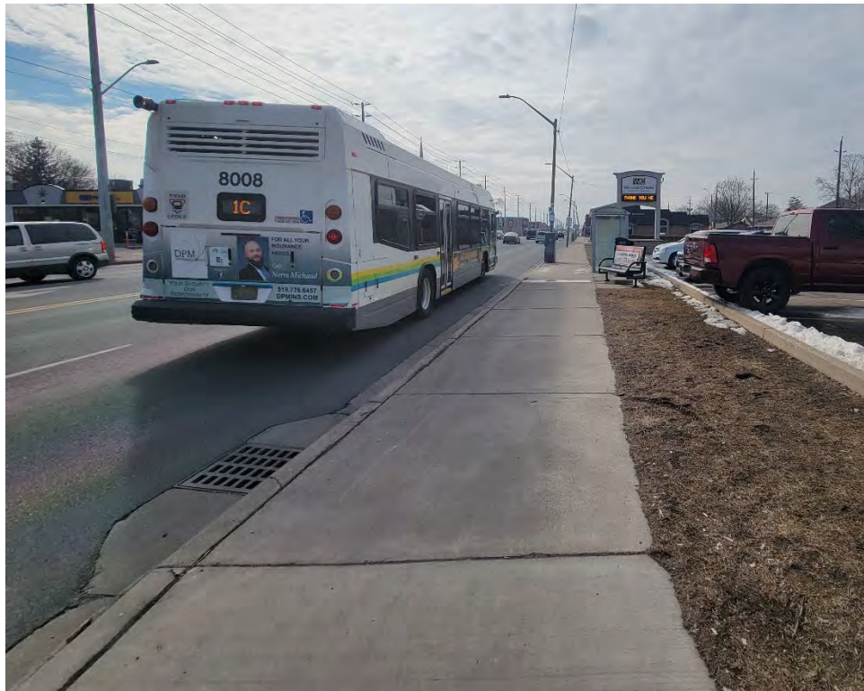
Figure 7 Example of Far-Side, In-Lane Bus Stop
