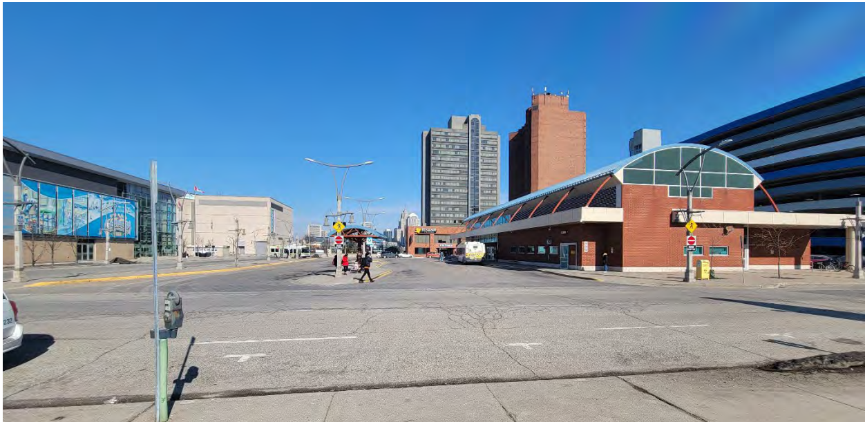
Figure 62 Windsor International Transit Terminal
