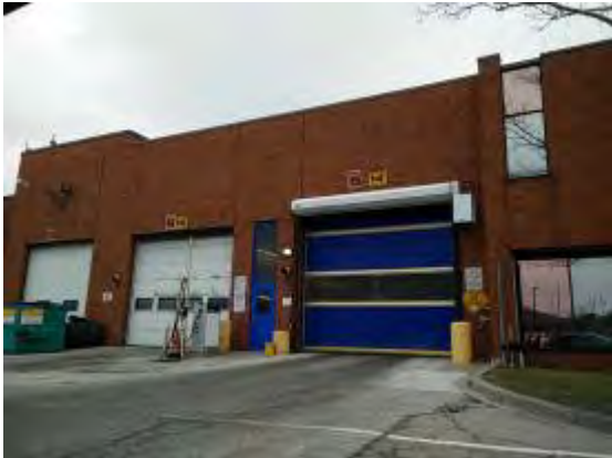
Large overhead garage doors for buses on west perimeter
