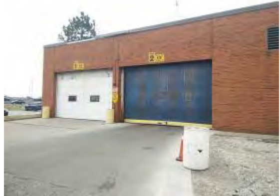
Large overhead garage doors on east perimeter
