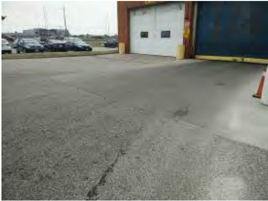
Concrete slab on grade before garage entrance
