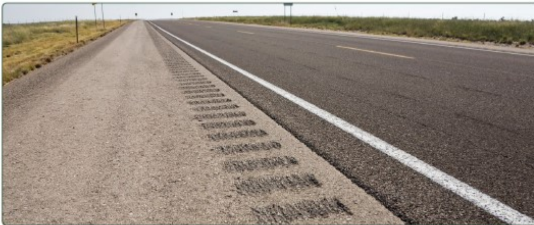
Figure 8: Pavement Edge Rumble Strip Example (Source: FHWA)
