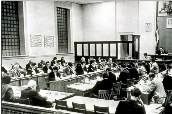
Interior Court Room 1975 showing the blocked in windows and lowered ceiling to accommodate air conditioning ducts (Court Auditorium – archival photo)
