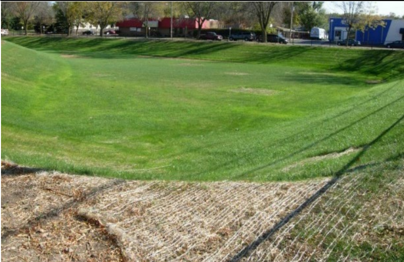
Option 2a and 2b - Dry Stormwater Pond
