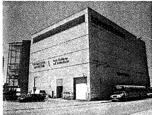
1F. South Side. Parking / Street View. - LED Channel Lettered Sign. - New Hardware & Lighting.
