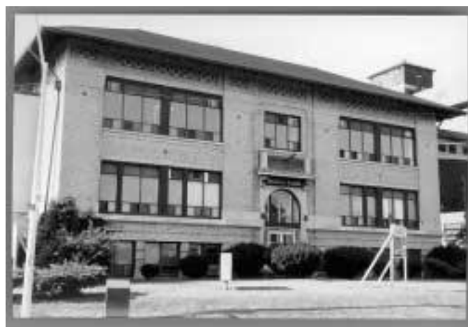
Ford City School, 1917 3177 Riverside Dr. E. (Demolished)
