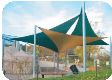
Figure 2: Constructed open air shade feature
