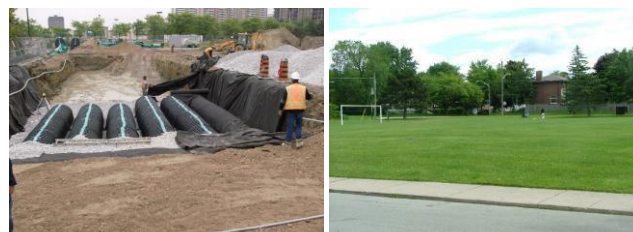
Figure 1: During and after construction (City of Toronto, 2009)
